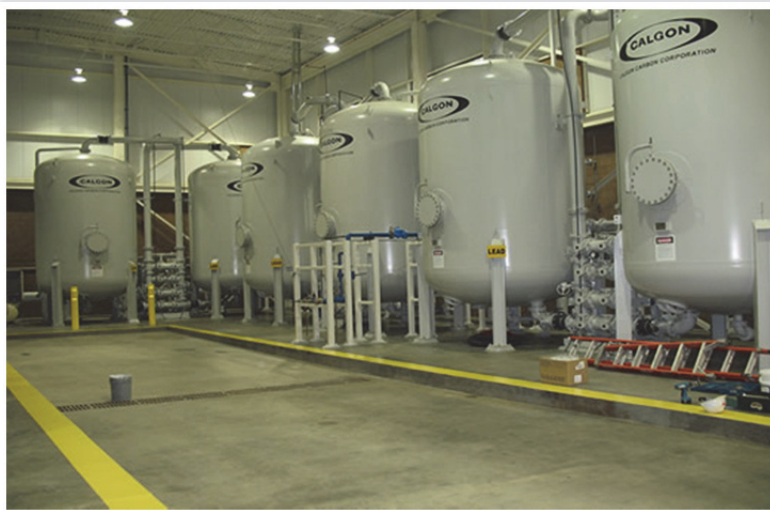
Source: Warrington Township A series of granular activated carbon filtration tanks used to treat contaminated groundwater in Warrington Township.
