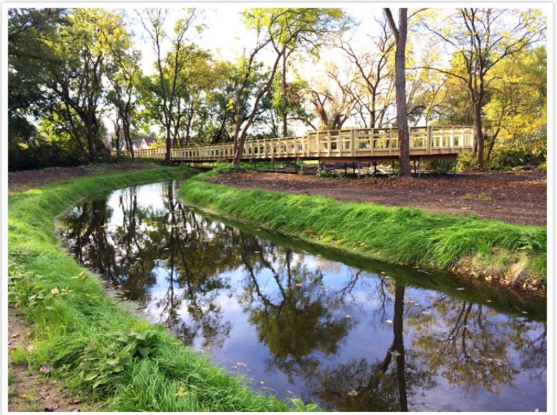
Source: CCMUA Baldwin's Run Daylighting is an example of a project undertaken by Camden SMART.
