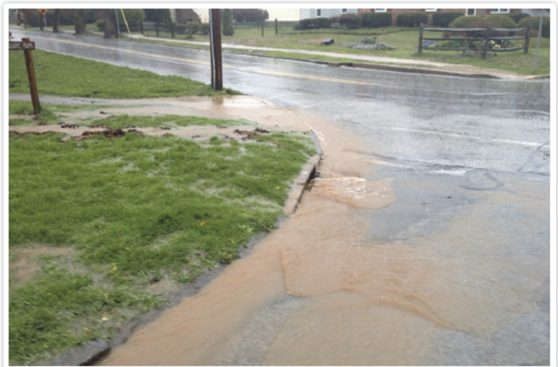
Source: West Chester Borough Public Meeting 2/2/17 Stormwater Fee Presentation This photo shows sediment-laden runoff in West Chester Borough.
