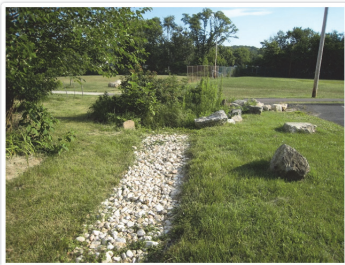
Source: Abington Township Abington Township's Parks and Recreational Department wanted to enlarge the crushed stone parking area near Roslyn Park and decided to add a rain garden on the down slope to assist with drainage and water quality.
