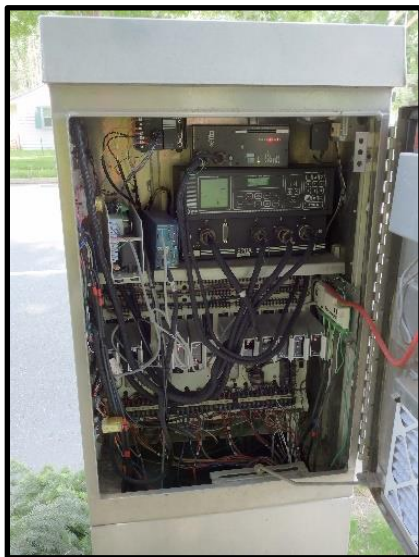
Photo 3: Multisonics 820A controller at Penn Lyle/Harris. Note presence of emergency preemption, NEMA monitor, and Autoscope interface. Monitor is placed on its side as space is limited in this cabinet.
