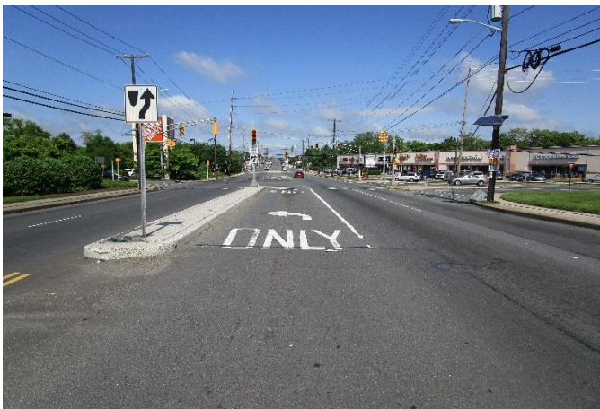
Photo 1: Looking NB on North Olden Avenue at Artie Parkway/Home Depot Driveway
