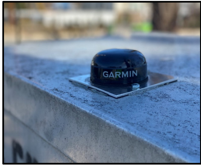
Photo 4: GPS Enabled Controller Cabinet
