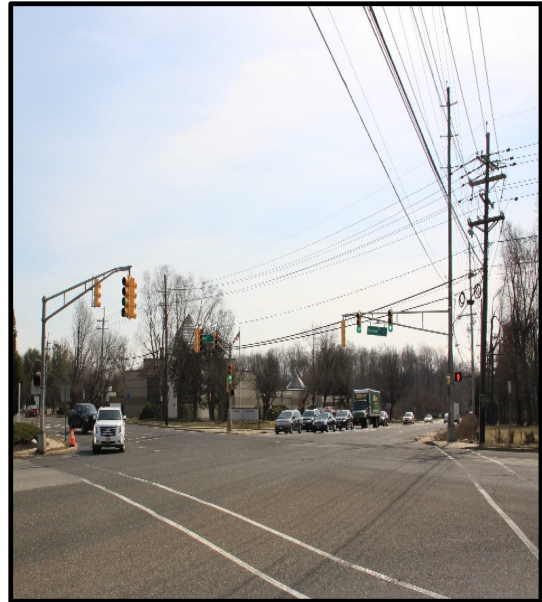
Photo 1: Kresson Road (CR 671) and Springdale Road (CR 673)
