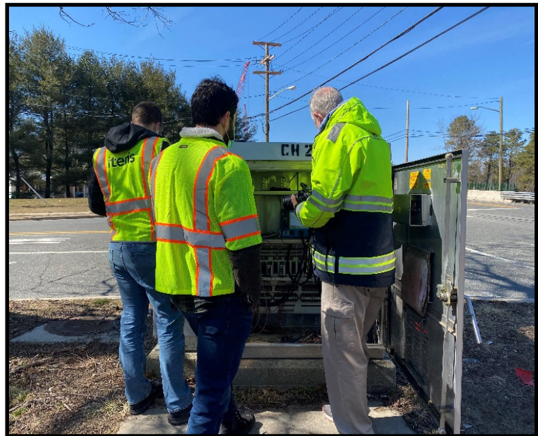
Photo 3: New Signal Timings Installed at Browning Lane
