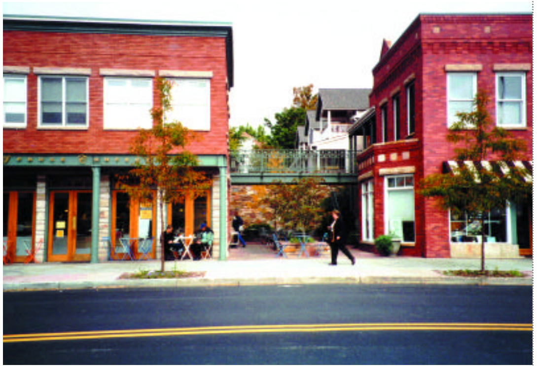
The buildings of the Eighth and Pearl mixed-use development in Boulder, Colorado, echo the character of the surrounding neighborhood. Retail and office space occupy the front of the complex, attractive townhomes and hidden parking are attached and transit is nearby.
