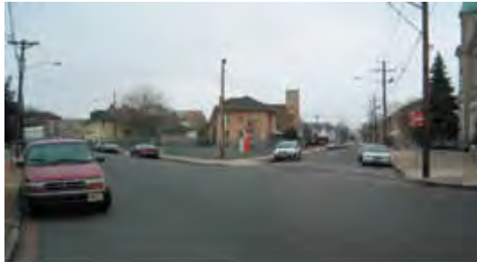
Photograph of Cass Street "before"
