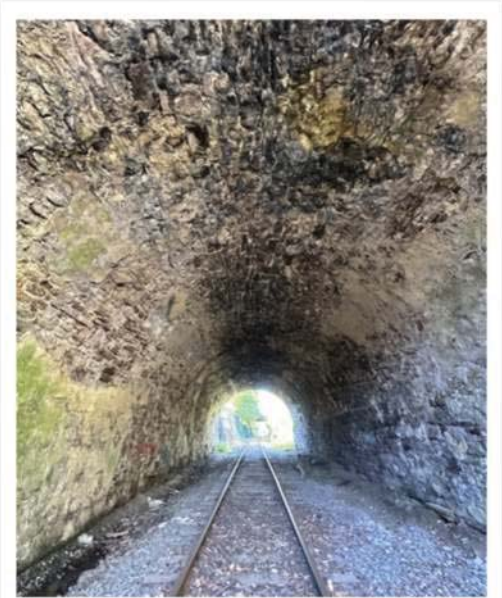
Bordentown Stone Arch Bridge (11/2022)
