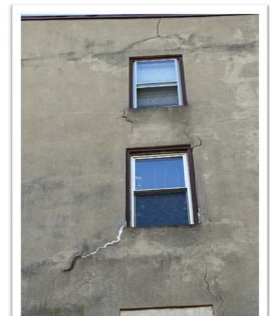
Existing three story building adjacent to bridge showing vibration / settlement sensitivity.
