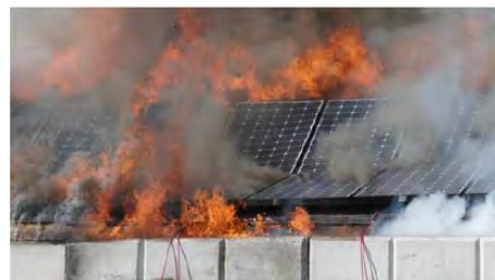
Figure 103 Roof and modules collapsing
