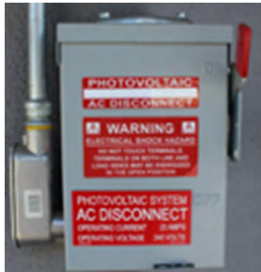
AC Disconnect Switch
