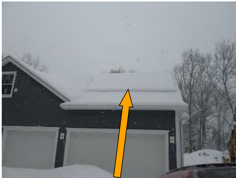
Array covered entirely in snow.
