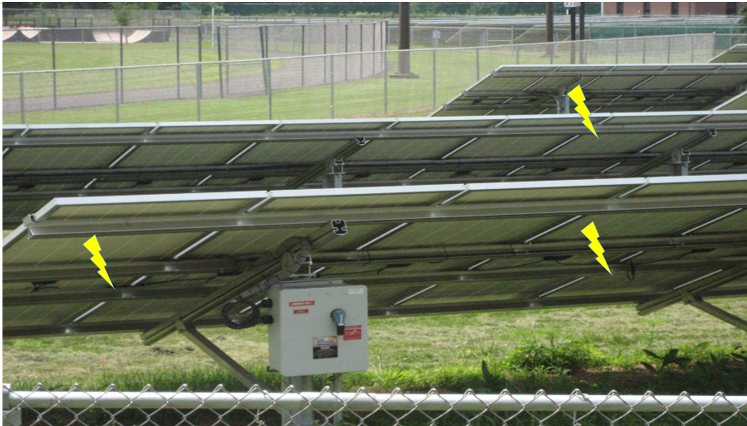
Ground-mount array with DC combiner/disconnect. Array conductors remain energized if disconnect is opened “off.”
