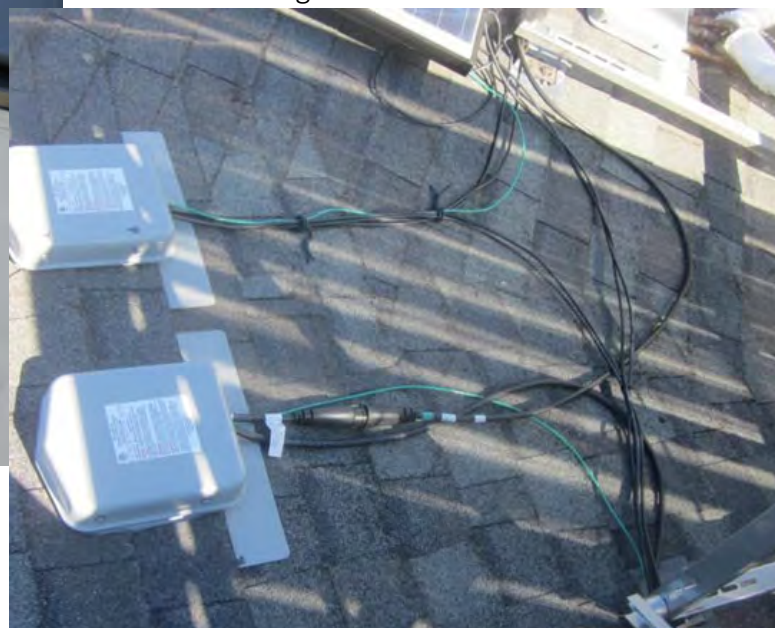
Poor wire management leads to additional hazards.
