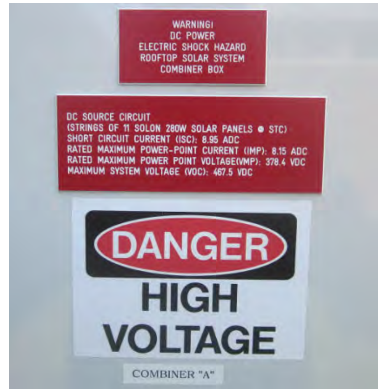
Maintenance label showing DC system properties.
