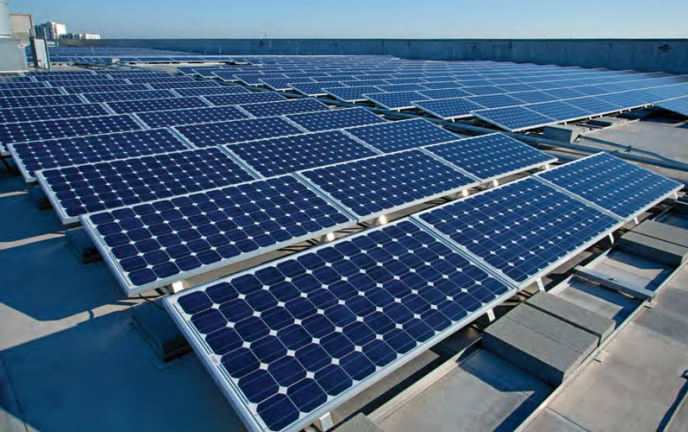
Roof Mount Commercial
