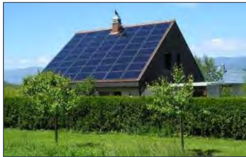
Solar Photovoltaic (PV)
