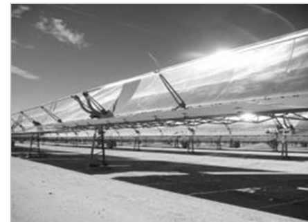
Concentrated Solar Power
