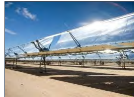
Concentrated Solar Power
