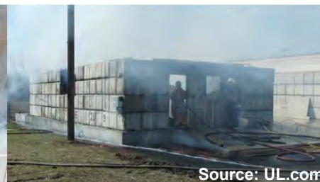
Figure 104 Roof collapsed -fire extinguished
