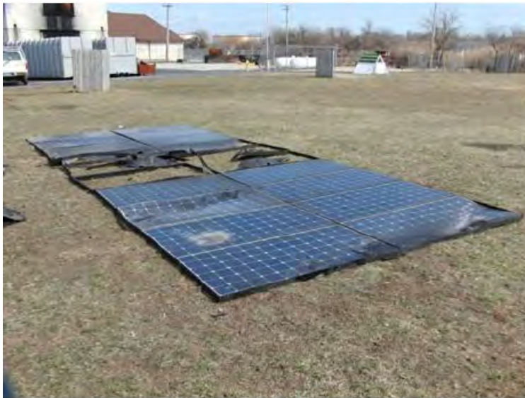
Figure 113 Post fire, front surface
