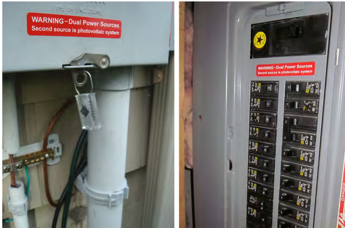
Warning label indicating multiple sources of power present.
