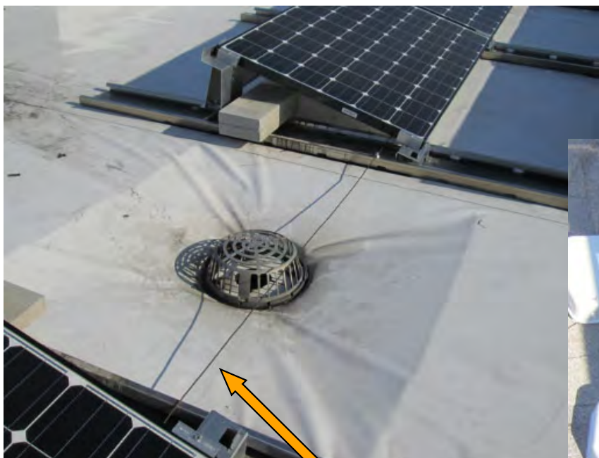
Be aware of conduit and conductors flat rooftops.
