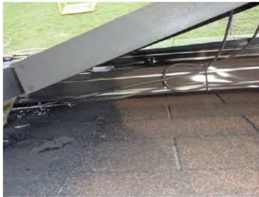
Figure 184 Looking under module for dangers
