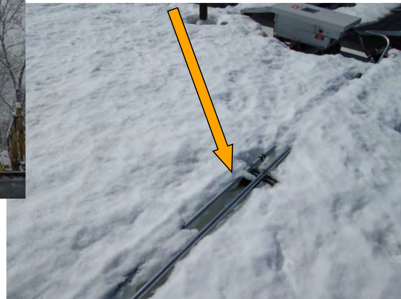
Rooftop conduits buried in snow.
