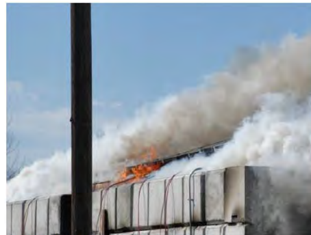
Figure 101 Open flames on roof
