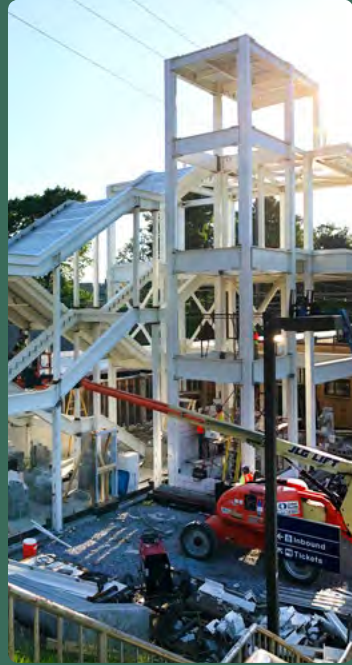
Paoli Train Station Construction Photo by Meijun Liu, Transportation Engineer, Office of Corridor Planning
