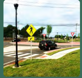
CR528/660 Roundabout, Burlington County, New Jersey Photo by Kwan Hui, Manager, NJ Capital Programs
