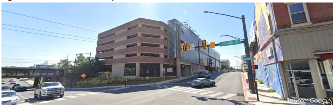
Figure 21: Norristown Transportation Center
