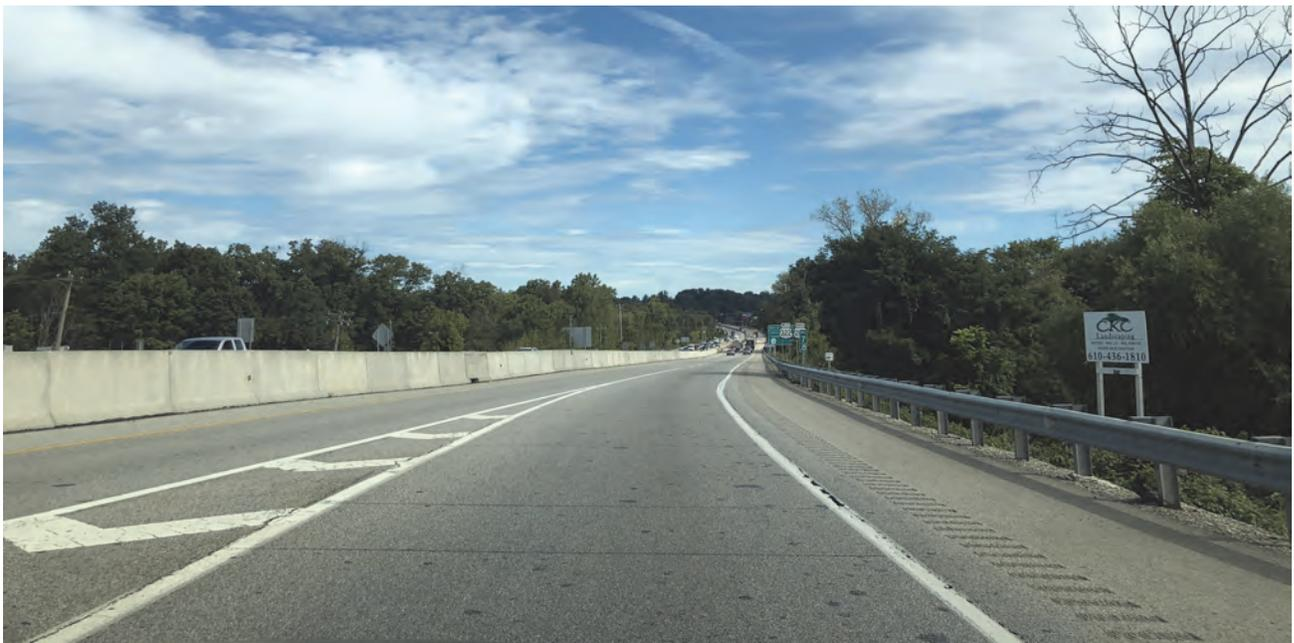
*At the top of the ramp, US 202 NB traffic flows freely into the right lane, and traffic merging from High Street flows freely into the left lane. Only about 250 to 300 vehicles merge from High Street, compared to almost 2,000 vehicles that are continuing NB from US 202. Nevertheless, both movements are currently given the same priority. Source: DVRPC, 2018*
