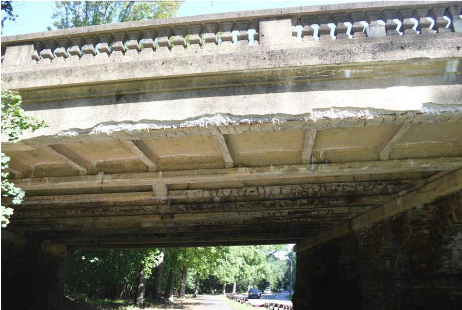
*Rebar pokes out of the underside of the functionally obsolete 65th Street Bridge above the Cobbs Creek Trail, September 2017.*
