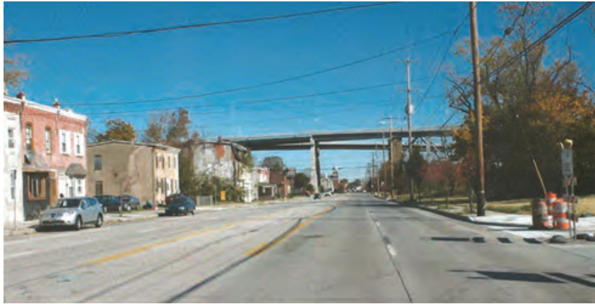
View looking east on PA Route 291 toward the US 322 off-ramp. Source: Oak Valley Design.
