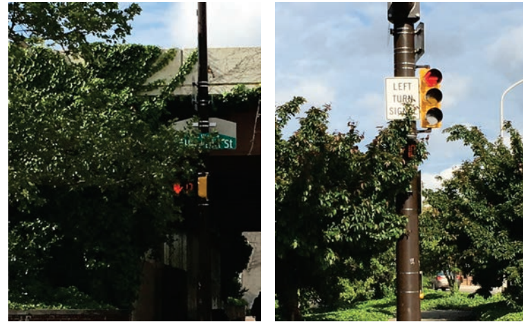
Figure 8: Tree Branches Covering the Signal Heads
