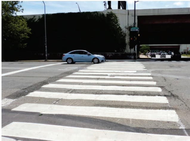
Figure 7: Long Crossing Distance on Callowhill Street
