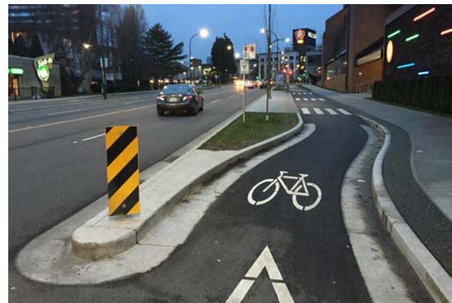
Figure 64 | Vancouver: Cornwall Avenue at Cypress Street
