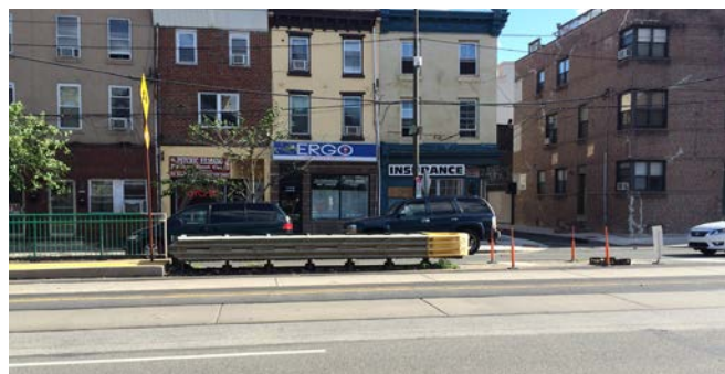
Figure 37 | A crash attenuator at a Route 15 trolley stop
