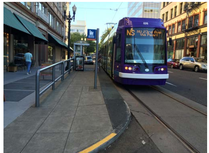
Figure 56 | Curb extension: Portland Streetcar
