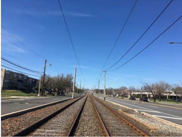
Figure 14 | Island Avenue near 76th Street
