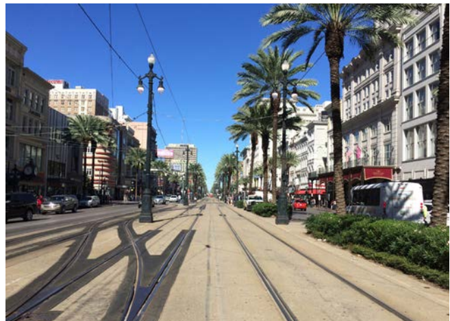
Figure 83 | New Orleans: Canal Street
