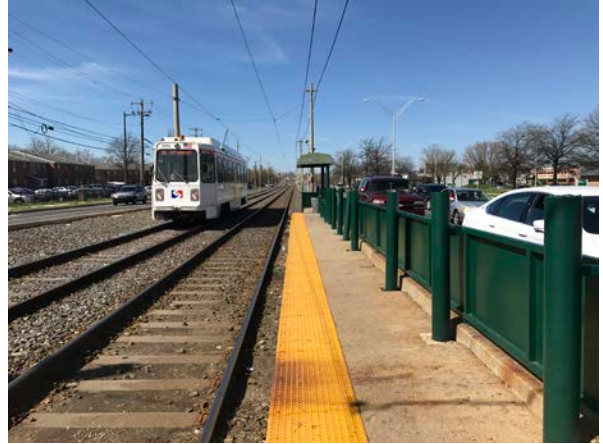
Figure 15 | Island Avenue & Lindbergh Boulevard
