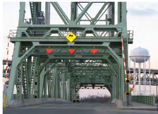
This bridge is located between Constitution Avenue and Langley Avenue in the Navy Yard. It leads to the 26th Street entrance to the Navy Yard.
