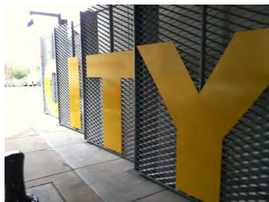
Phase I of the Race Street Connector is completed; Phase II will be finished in fall 2012.
