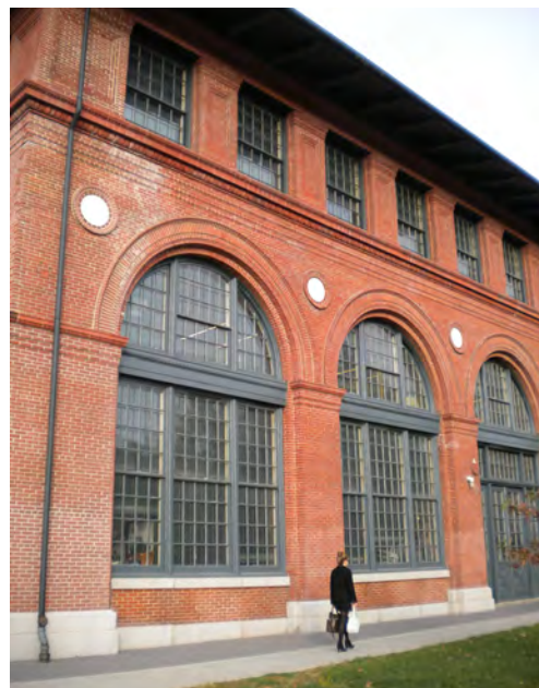
Several of the buildings at the Navy Yard will receive energy efficiency upgrades as part of the GPIC’s Energy Innovation Hub for Energy-Efficient Buildings.
