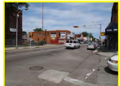
Pedestrian heads misaligned at Chase St crossing Mt. Ephraim Ave to the school, and over Chase St. Pavement markings are missing.
