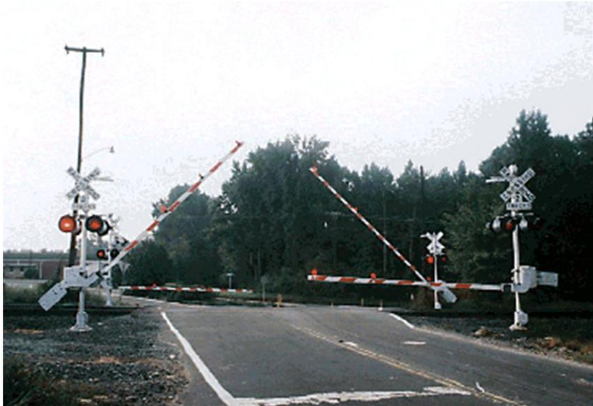
*Left: A four-quadrant gate in North Carolina (note: the gates to the entrances are already closed, but the gates for the exits are in the process of closing). (Source: North Carolina Department of Transportation)*
