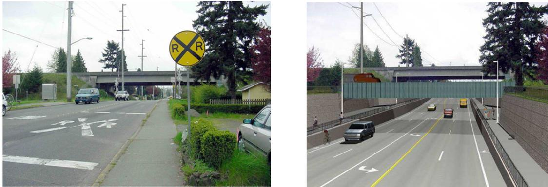
Left: Present at-grade conditions at M Street in Auburn, WA. Right: A rendering of a planned roadway tunnel under the rail line in Auburn, WA. (Source: Puget Sound Regional Council)
