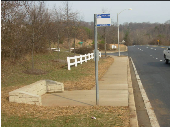
Knee wall and concrete pad at bus stop (Source: Montgomery County, MD 2011)
