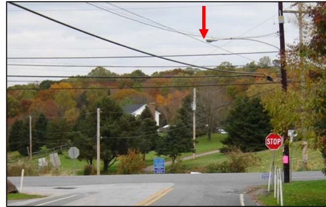
Rural intersection lighting.
