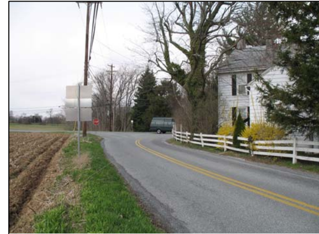
Access to private residences is too close to several intersections.
