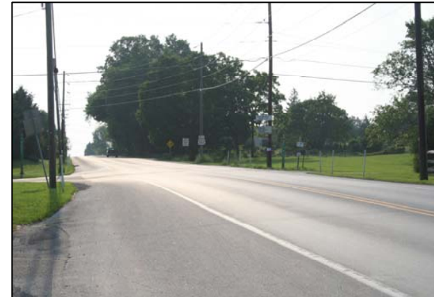
Intersection of Birdell Road and US 322
