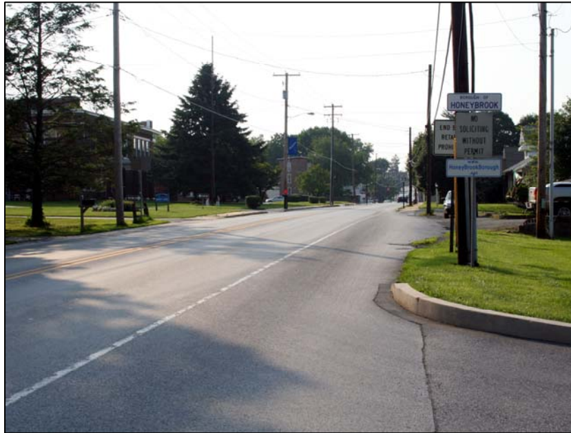
Figure 11: Before and After Gateway into Honey Brook Borough
