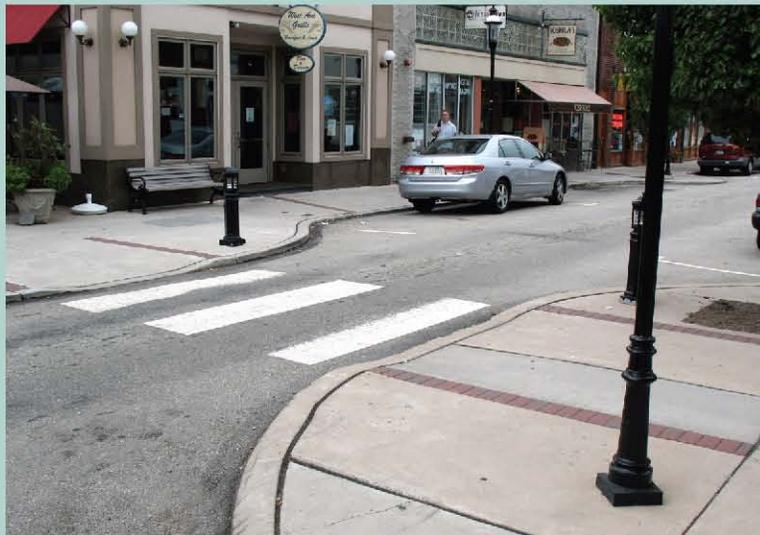
*Jenkintown Borough in Montgomery County, PA installed curb bumpouts as a traffic calming measure, forcing traffic to slow down. In addition to the calming benefits, the bumpouts shorten the pedestrian crossings and create contained streetside parking. Source: DVRPC*
