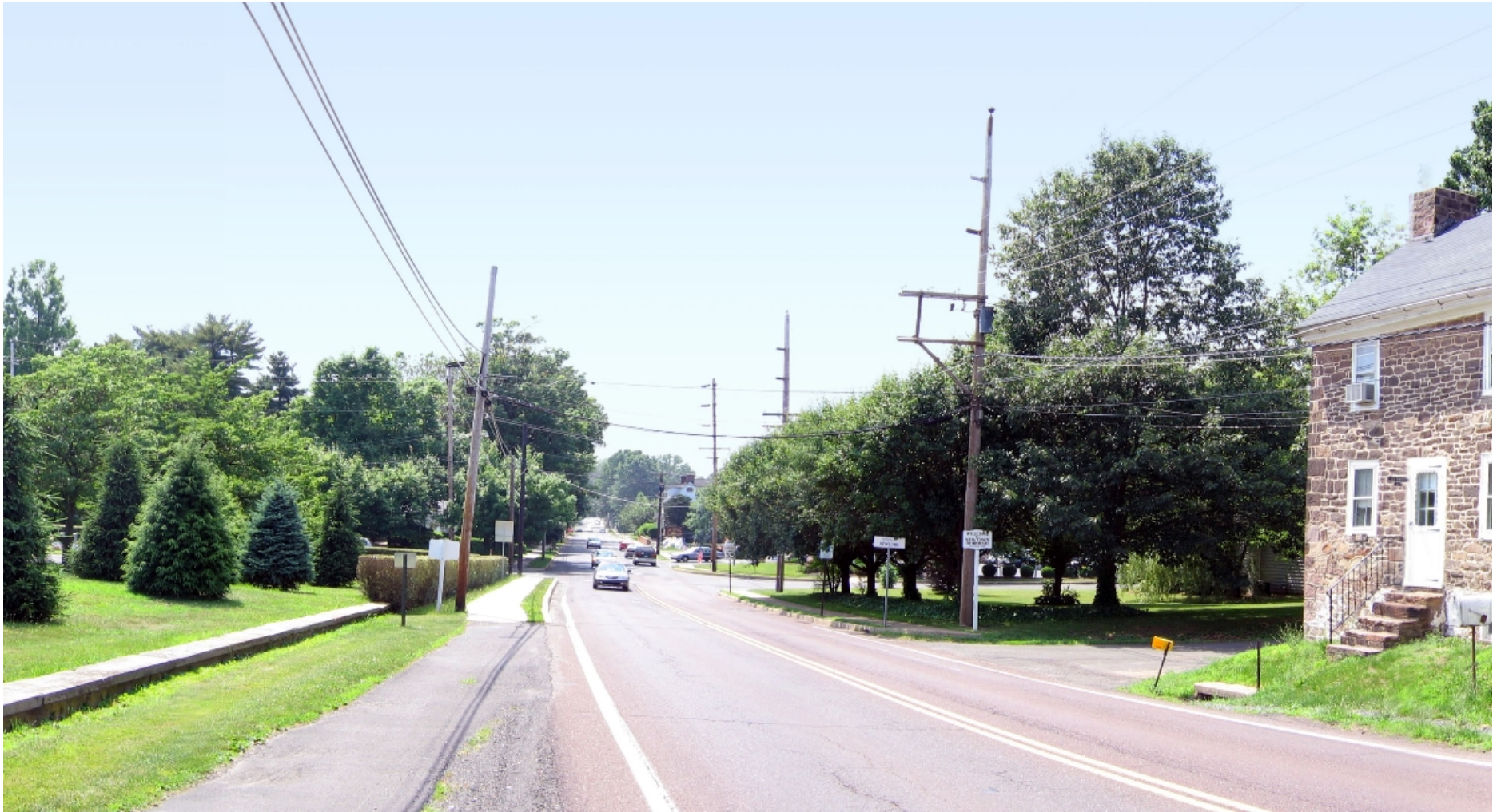
Figure 2: Existing Conditions on Washington at Elm. Spring 2005. Source: DVRPC.
