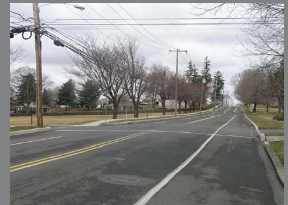
Lincoln Avenue is a minor collector street in Newtown Borough.
