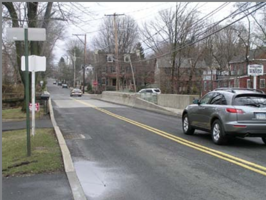
Jefferson Street heading eastbound travels past many older homes in the Borough.
