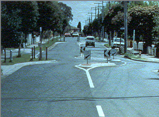
A chicane is an S-shaped curve within an otherwise straight roadway, designed to slow drivers down. They are appropriate only at mid-block. The City of Chester uses a chicane in its downtown shopping district, one of the few in the Philadelphia region. Photo by ITE.
