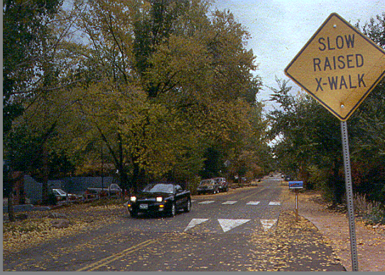
A speed table three to four inches high reduces speed. Fire departments prefer speed tables over speed humps. Photo by ITE.
