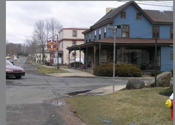
A traffic signal has been installed at the intersection of Sycamore and Jefferson as part of the Sycamore Street reconstruction.
