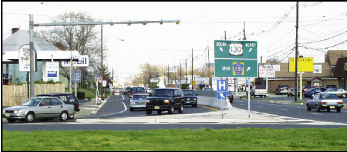
Figure 4: Looking at southbound US 130 entering the East Circle
