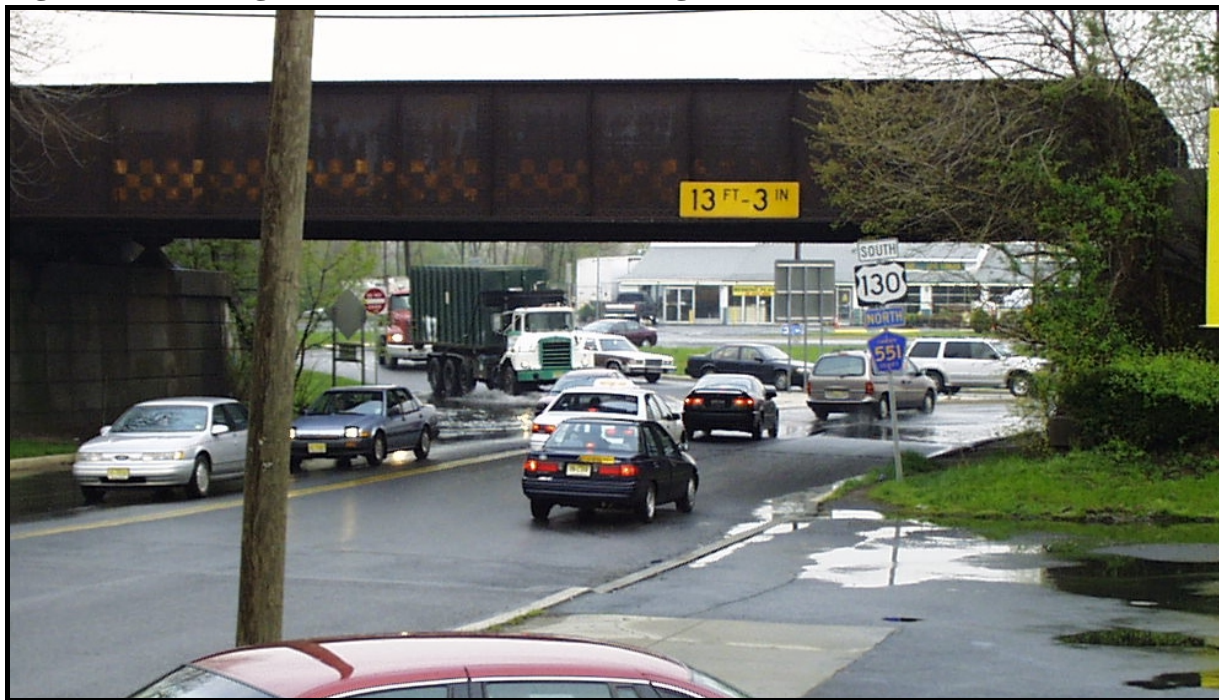
Figure 22: Looking Toward the West Circle along US 130 from the East Circle
