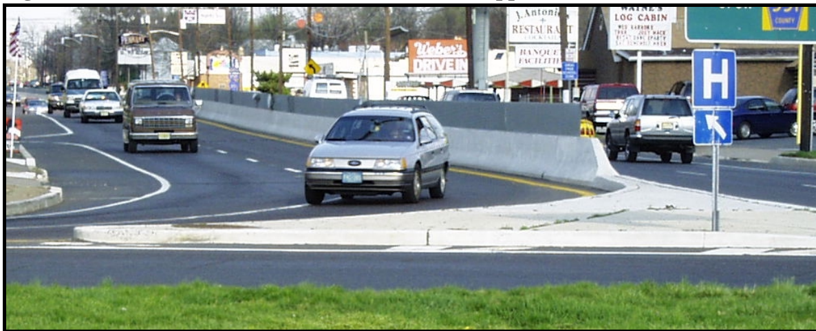
Figure 15: Concrete Island at Southbound US 130 Approach to the East Circle
