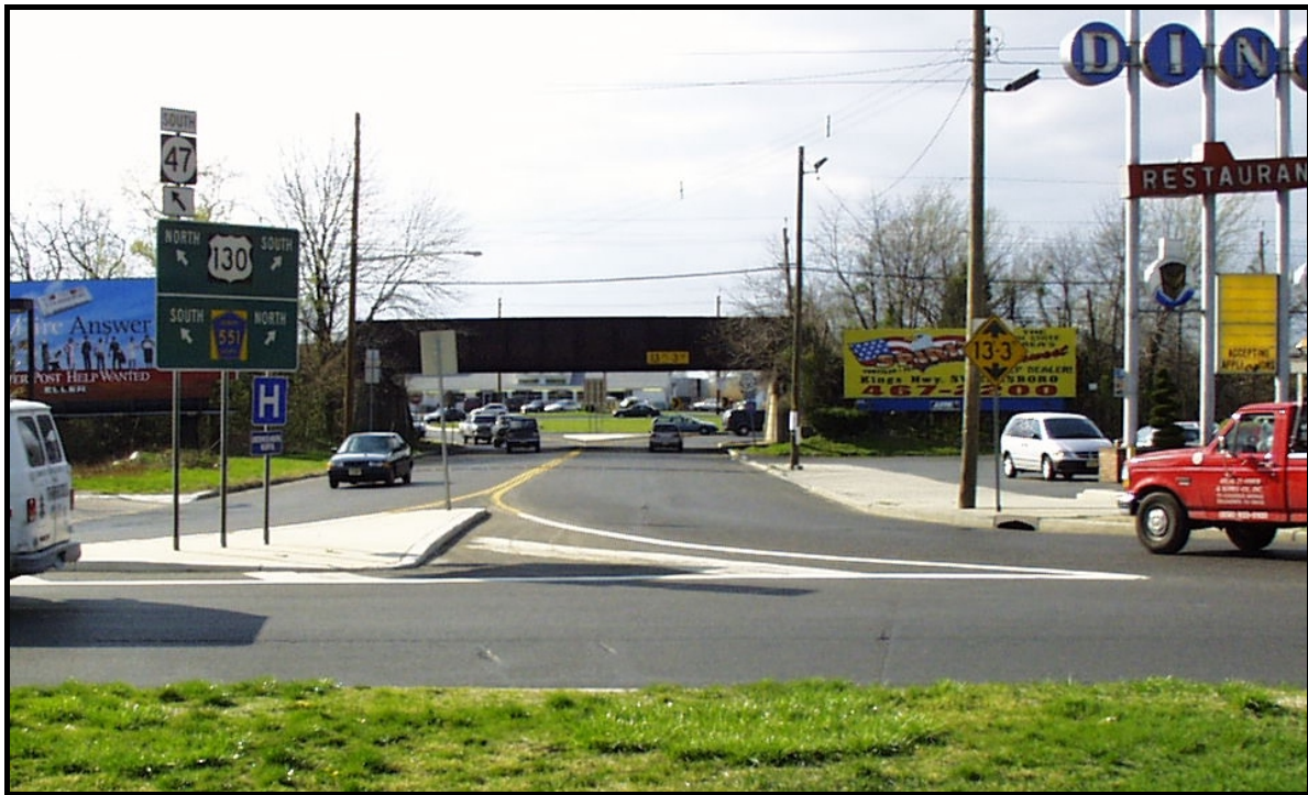
Figure 6: Looking Toward the West Circle along US 130 from the East Circle
