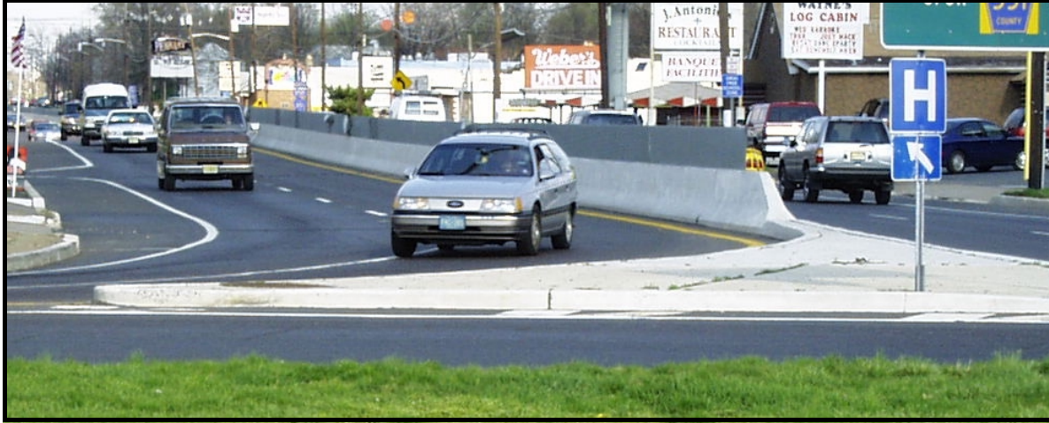
Figure 25: Looking at Concrete Island at US 130 at the East Circle
