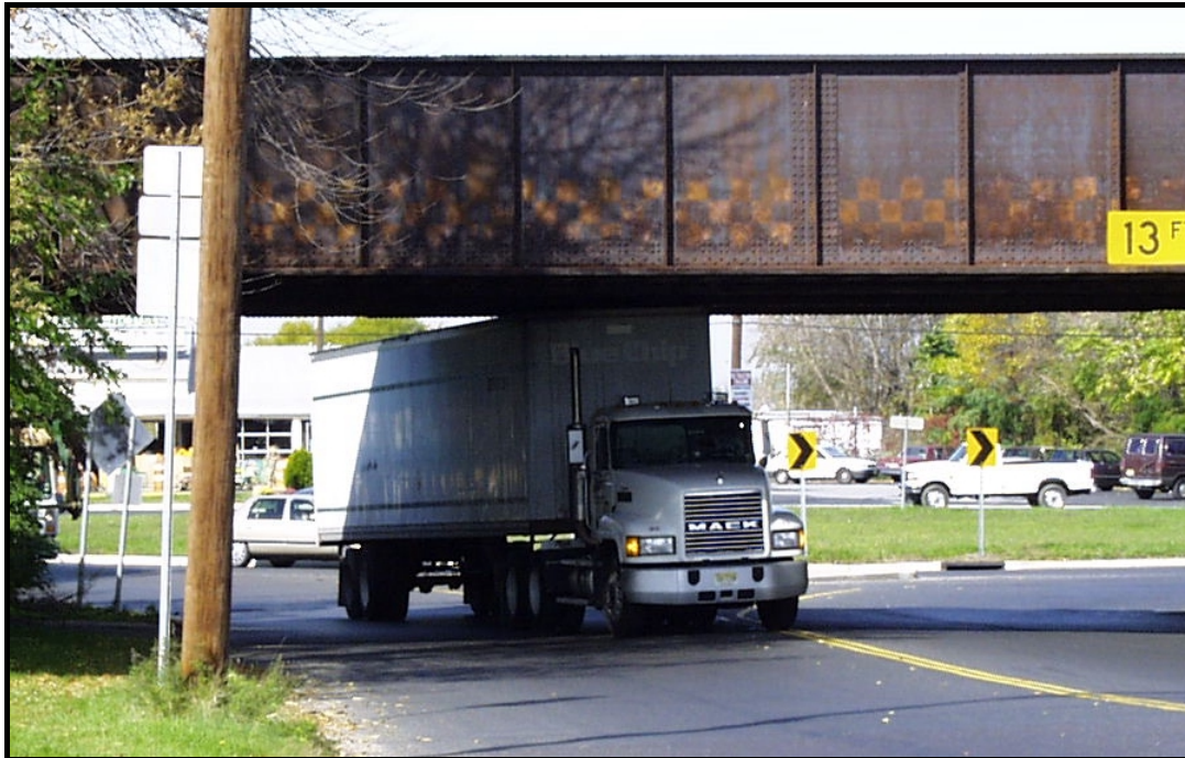
Figure 21: Conrail Railroad Bridge Between the East and West Circles
