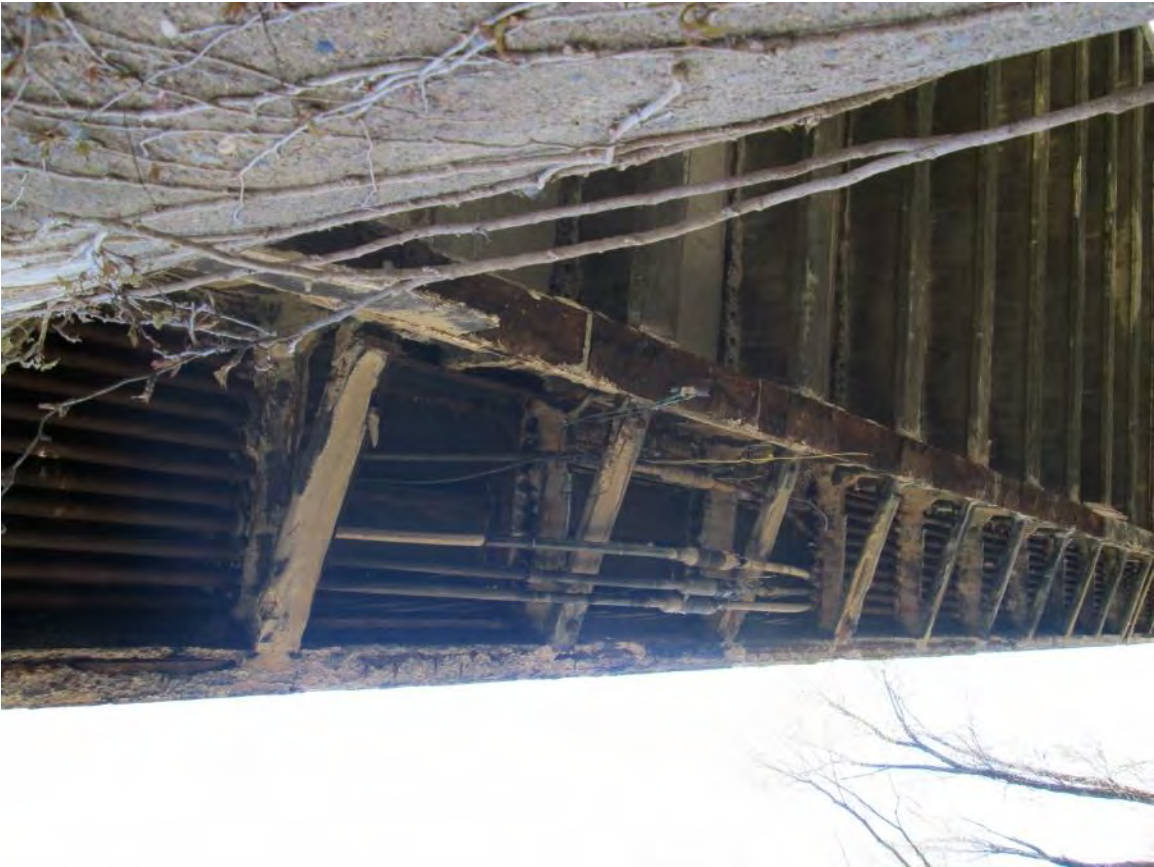
Figure 5 – Underside of sidewalk, showing 10 existing conduits
