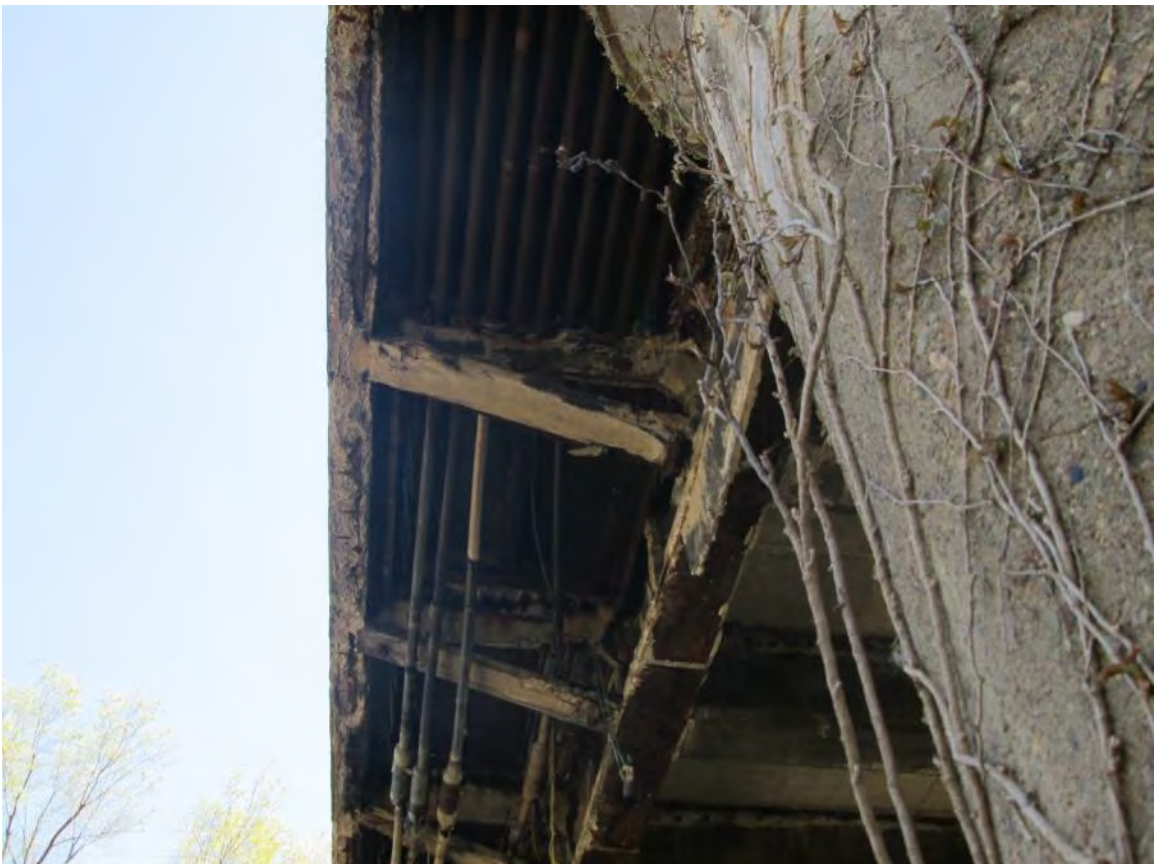
Figure 4 – Underside of sidewalk, showing 10 existing conduits
