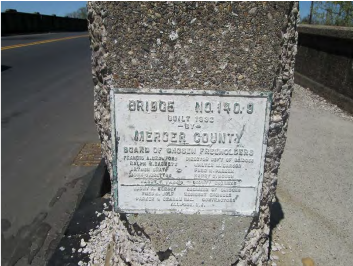
Figure 37 – Bridge Plaque along Lincoln Avenue westbound approach
