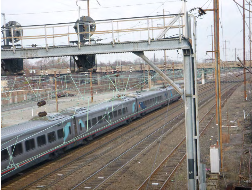
Plate 11: Lincoln Avenue Bridge, Northeast Corridor with bridge in background.
