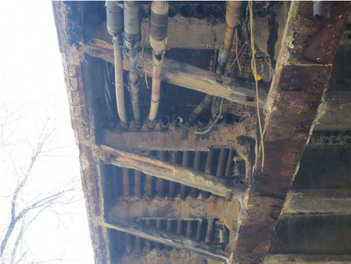
Figure 1 – Underside of sidewalk, showing 10 existing conduits
