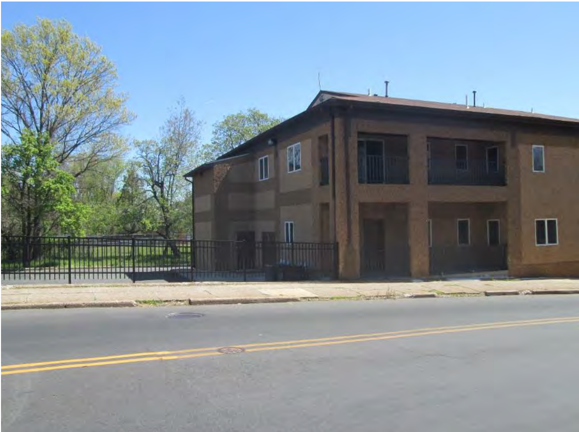
Figure 48 – Lincoln Avenue, looking north at Martin House
