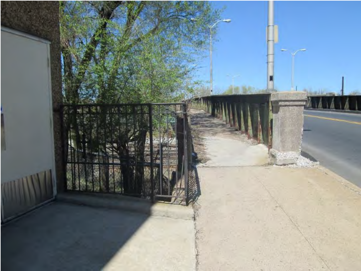
Figure 49 – Lincoln Avenue, looking northwest at sidewalk on south side of bridge
