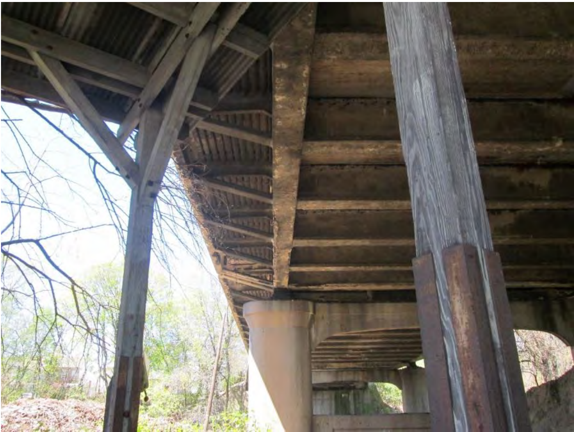
Figure 9 – Underside of south side sidewalk, looking west showing 10 existing telephone conduits
