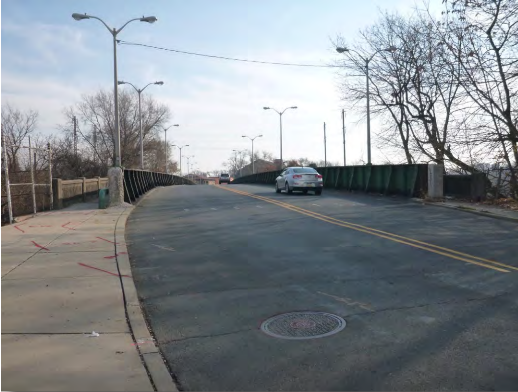
Plate 1: Lincoln Avenue Bridge (north end).
