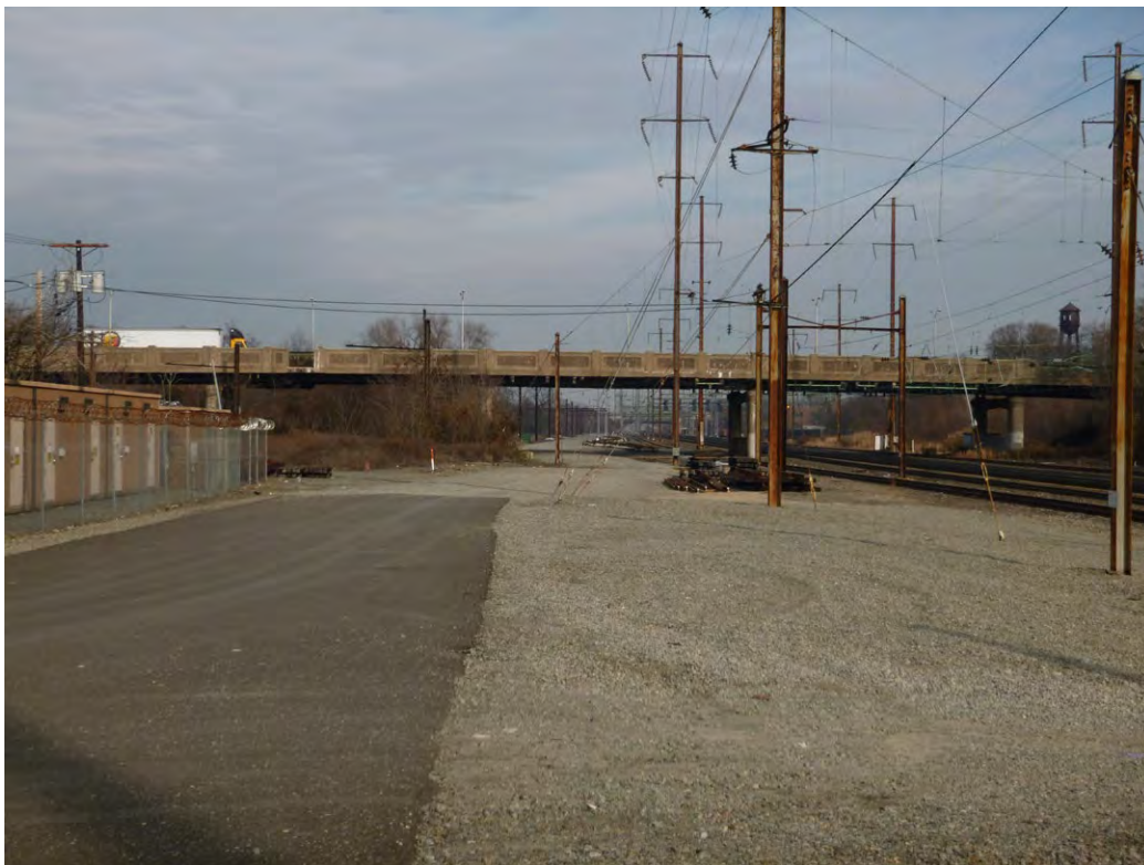
Plate 6: Lincoln Avenue Bridge, with North East Corridor tracks at right.
