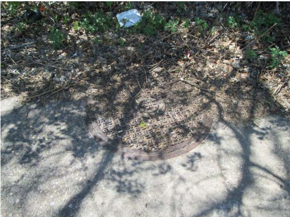
Figure 62 – Manhole in Sidewalk on South Side near Creekview Drive
