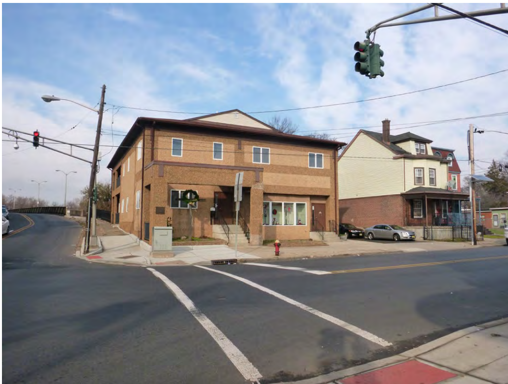
Plate 16: Lincoln Avenue Bridge, Chambersburg neighborhood, bridge (far left), 800 block East State Street (right).
