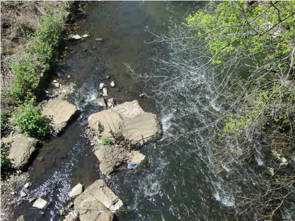
Figure 59 – Assunpink Creek, looking south showing concrete in waterway
