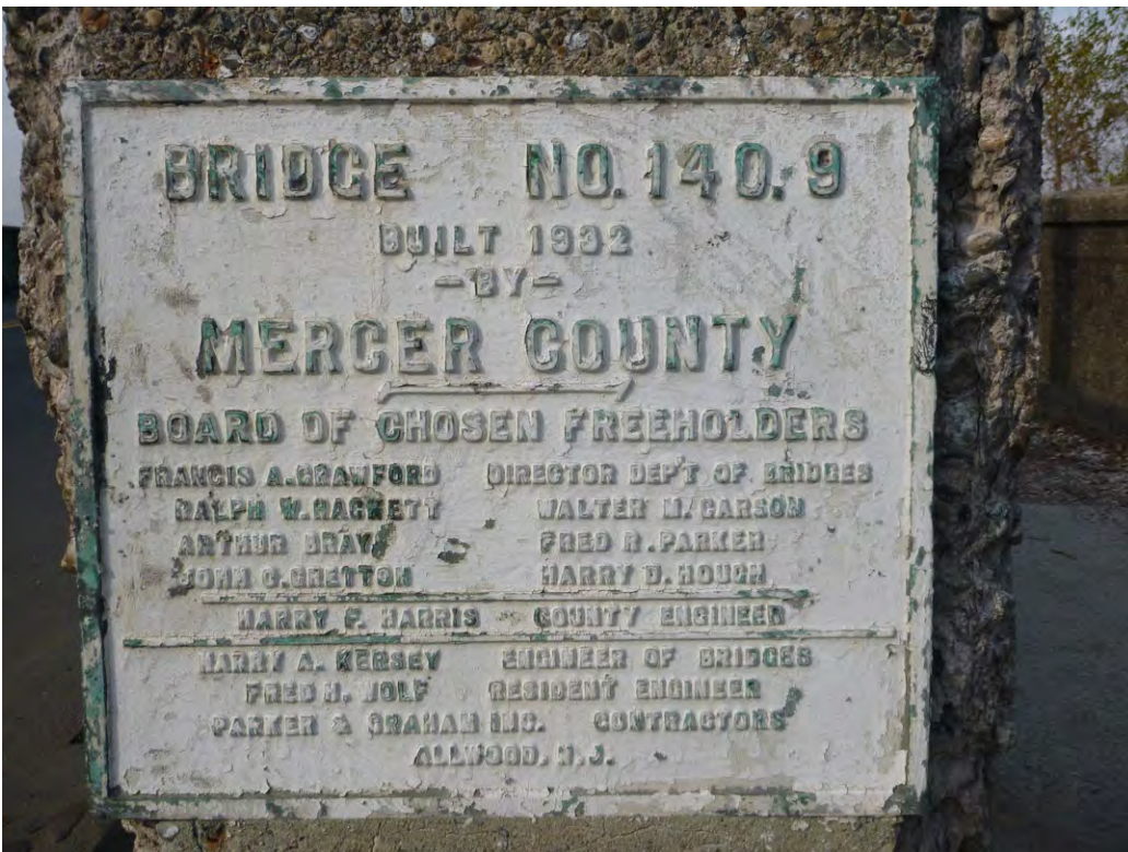
Plate 4: Lincoln Avenue Bridge (south end), plaque.
