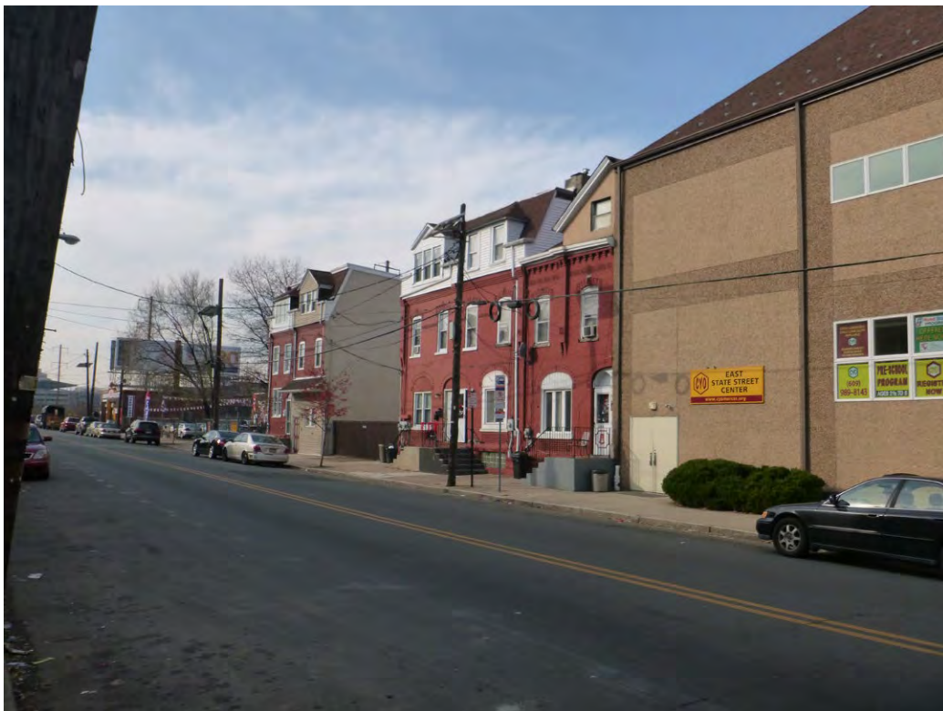
Plate 20: Lincoln Avenue Bridge, Chambersburg neighborhood, 700 block East State Street, north side.
