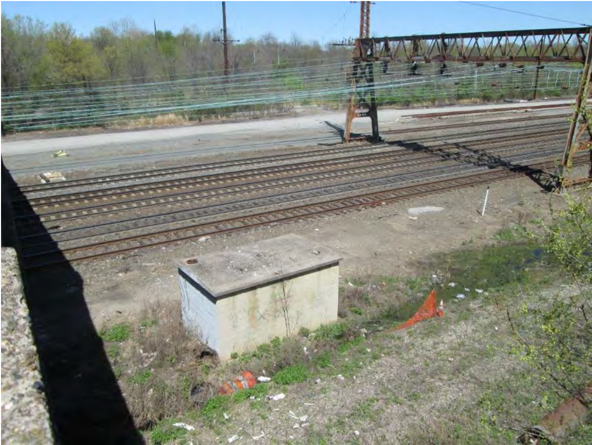
Figure 35 – NEC and Catenary Lines, looking northwest
