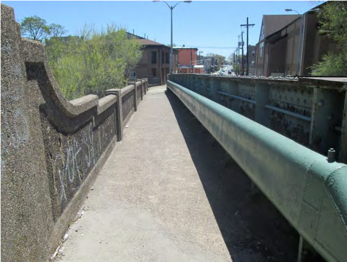
Figure 31 – Existing Gas Main Attached to North Side of Structure, looking southeast
