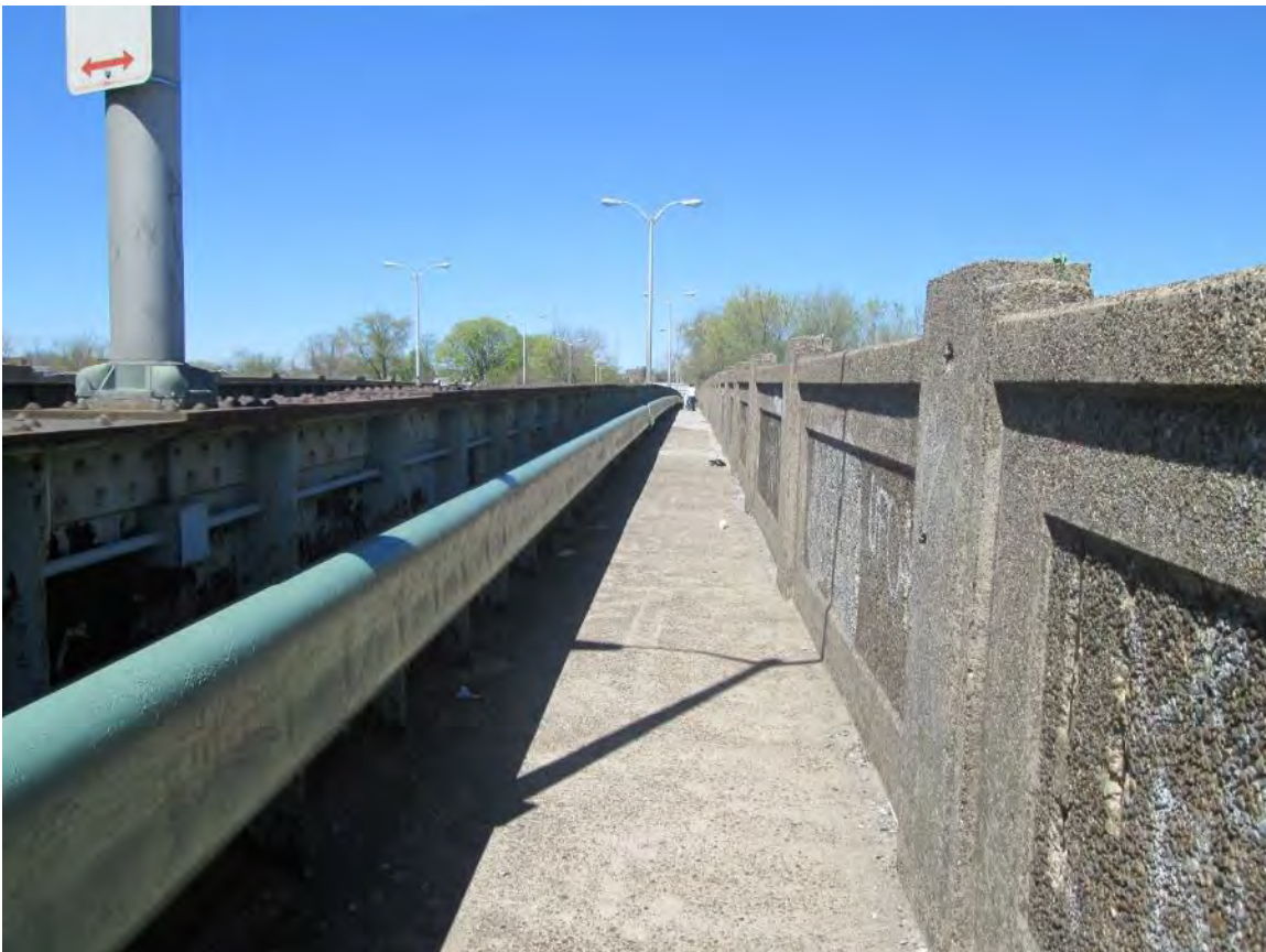
Figure 32 – Existing Gas Main Attached to North Side of Structure, looking northwest
