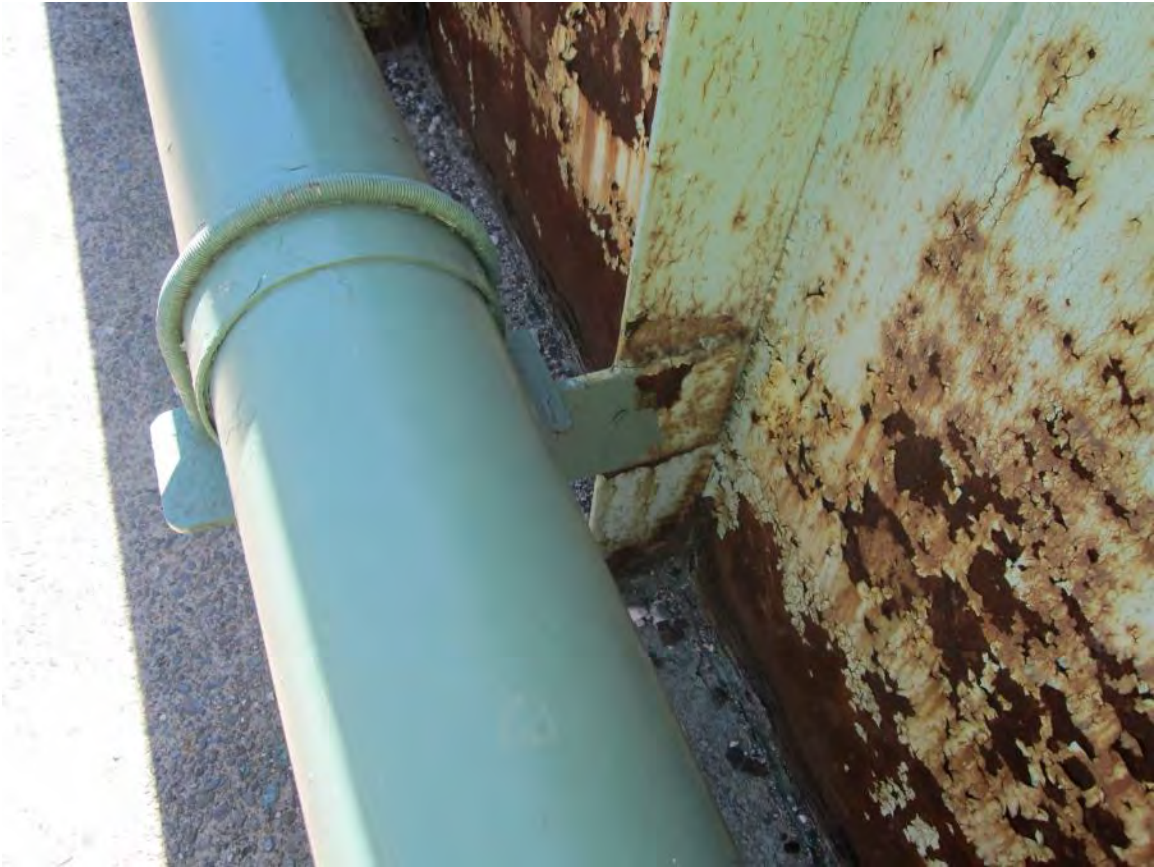
Figure 25 – Existing Gas Main Attached to North Side of Structure
