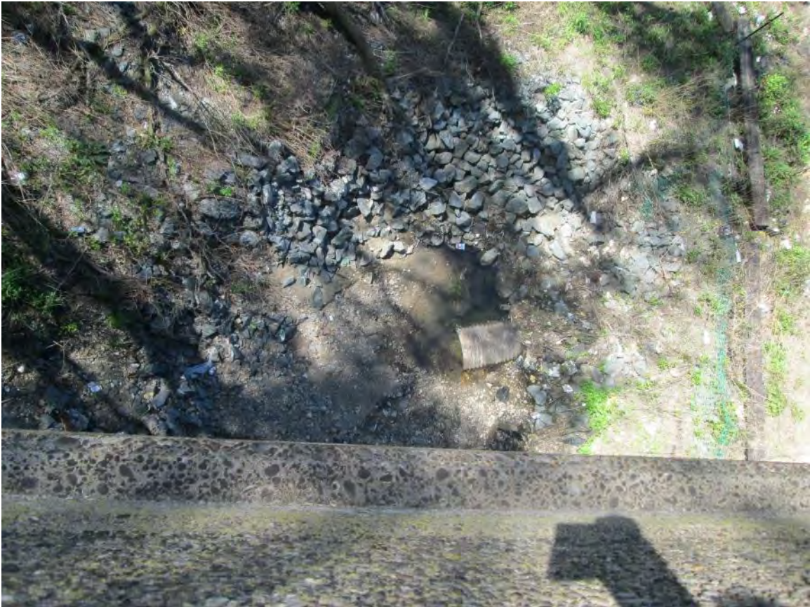
Figure 51 – Existing Corrugated Metal Pipe near Eastern Abutment
