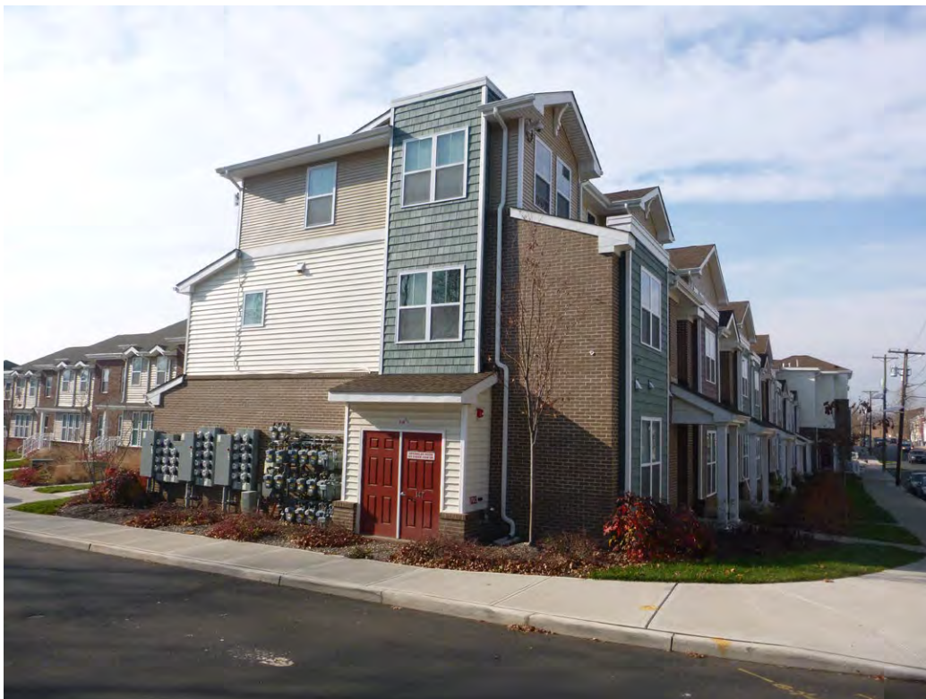
Plate 14: Lincoln Avenue Bridge, new housing on Lincoln Avenue, north end of bridge.
