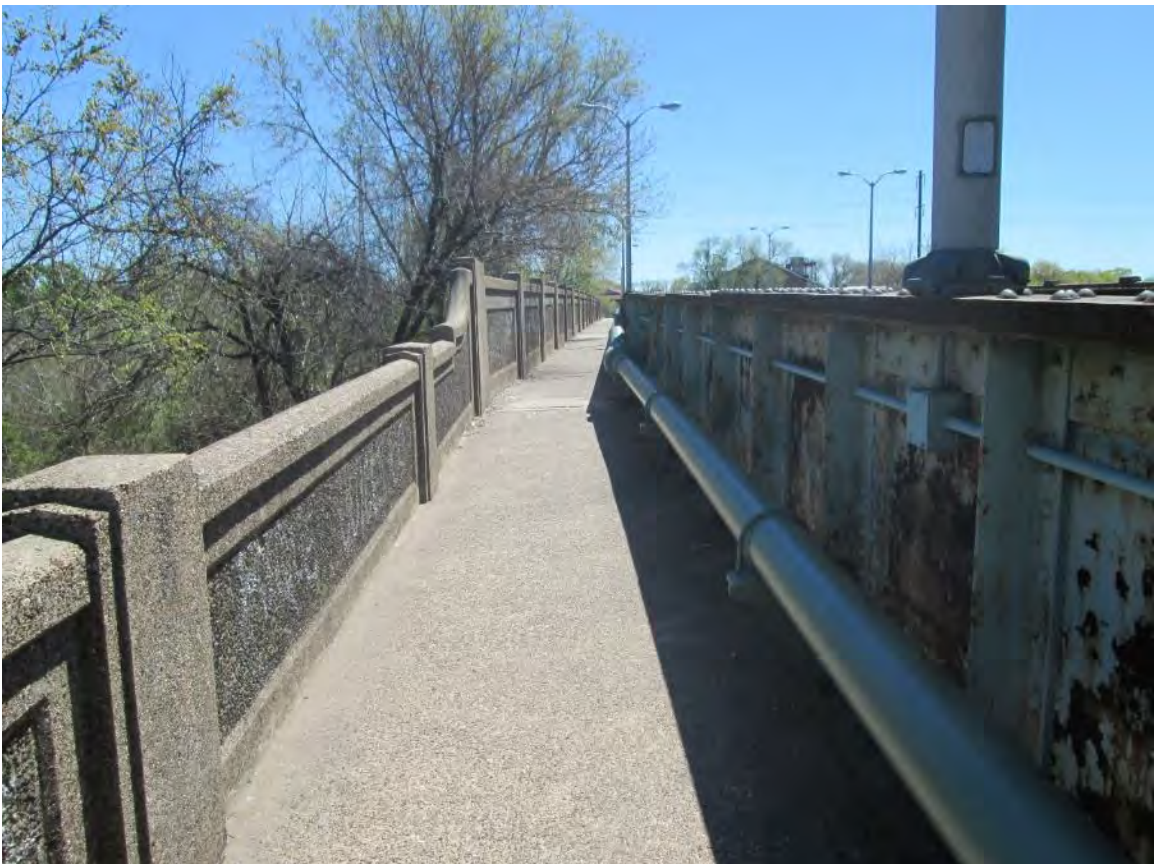
Figure 26 – Existing Gas Main Attached to North Side of Structure
