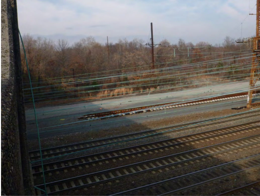
Plate 13: Lincoln Avenue Bridge, terrain and Northeast Corridor tracks in foreground, northeast of bridge.
