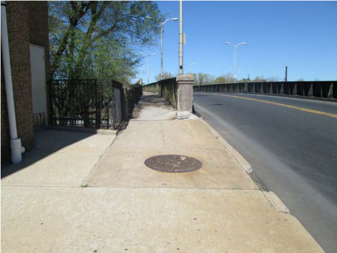
Figure 47 – Lincoln Avenue near E. State Street, showing junction box in sidewalk by CYO E. State Street Center
