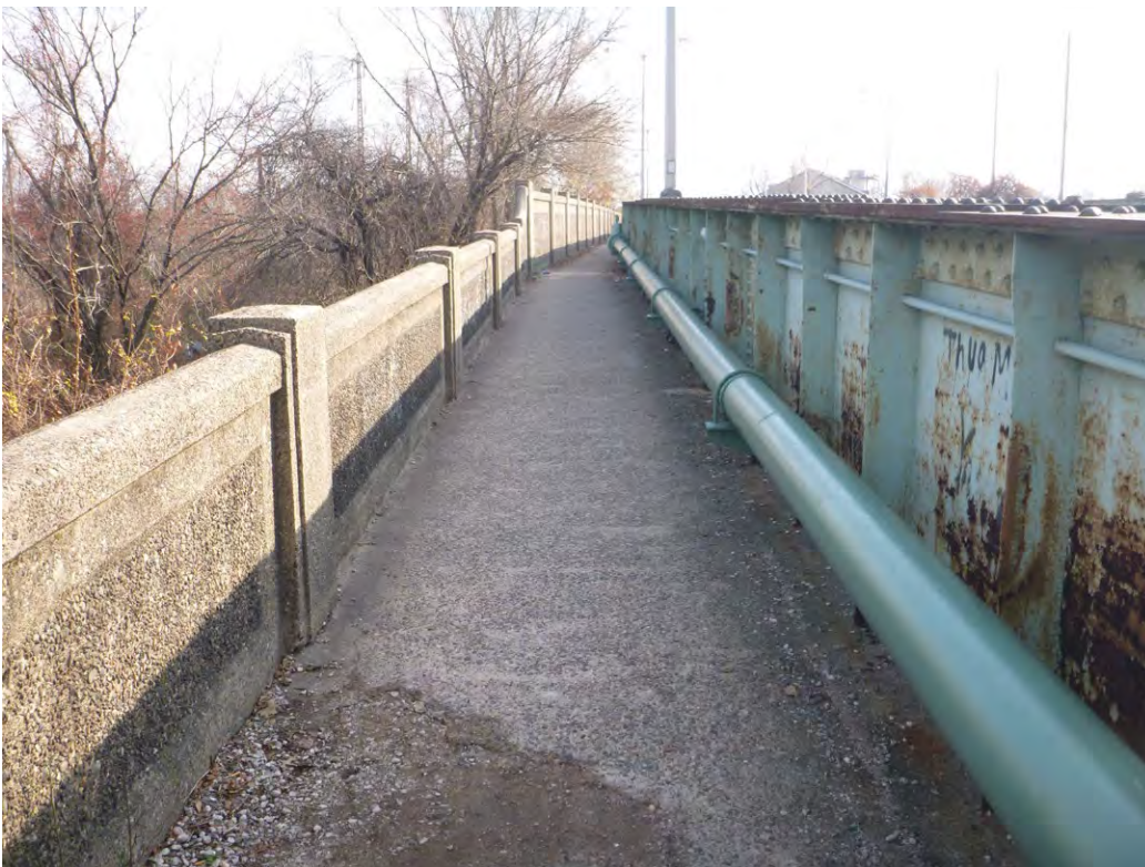
Plate 2: Lincoln Avenue Bridge (north end), east side walkway.
