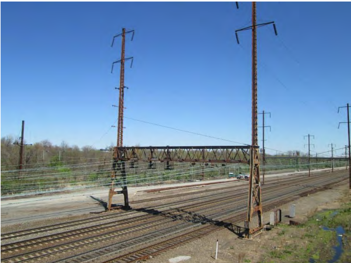
Figure 34 – Northeast Corridor (NEC), Catenary Lines and Transmission Lines, looking north
