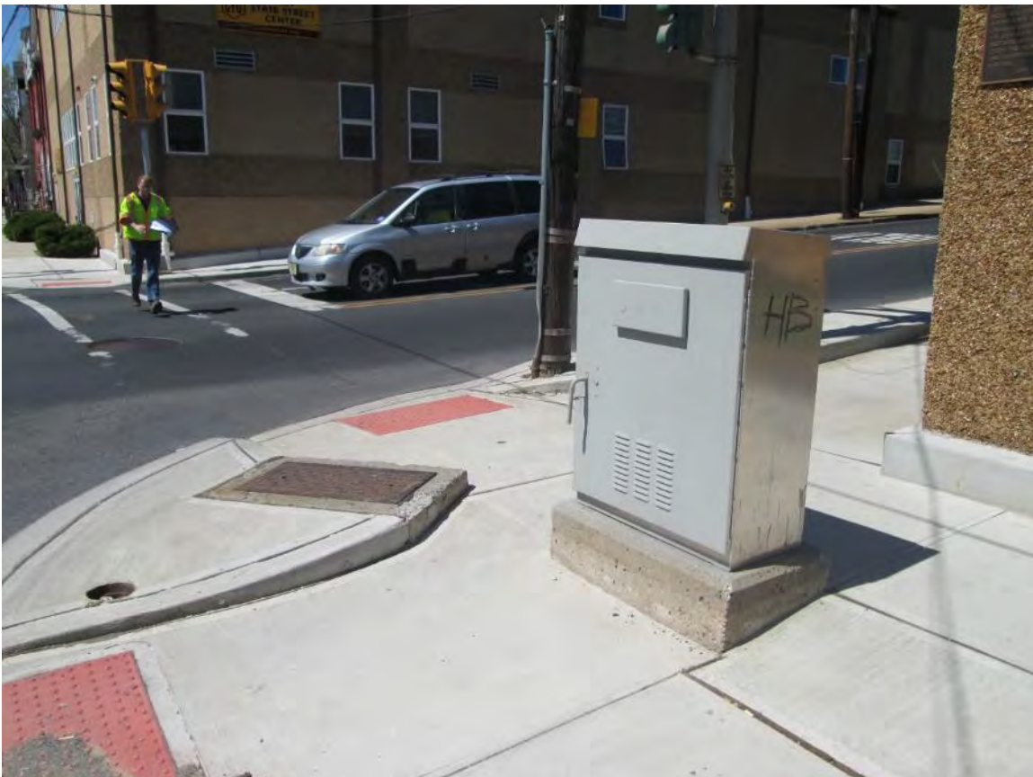
Figure 40 – Northwest quadrant of Lincoln Avenue and E. State Street, looking south showing curb ramps
