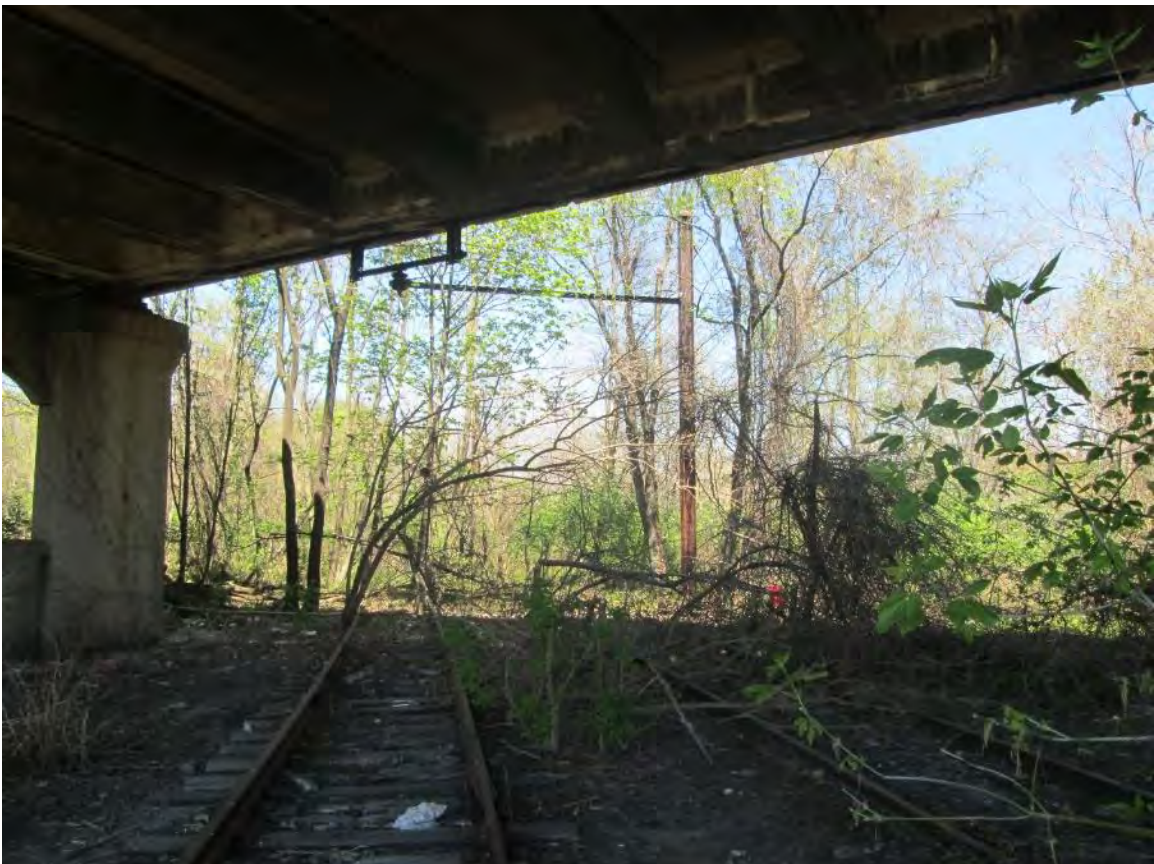
Figure 6 – Inactive NJ Transit Tracks, looking north
