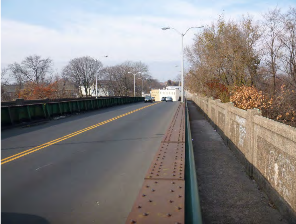
Plate 3: Lincoln Avenue Bridge, west side walkway and road bed.
