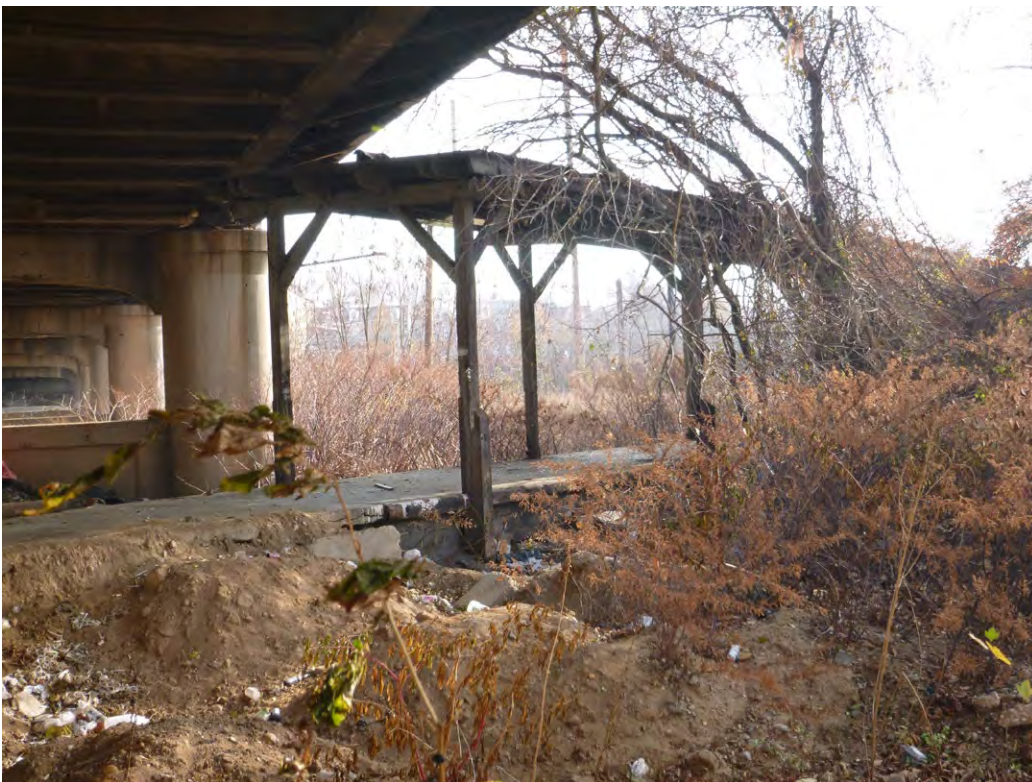
Plate 10: Lincoln Avenue Bridge, siding element, beneath/west of the bridge, showing platform on spur line.
