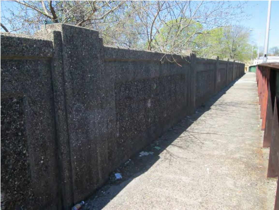
Figure 53 – Existing Parapet along Bridge (Typical)
