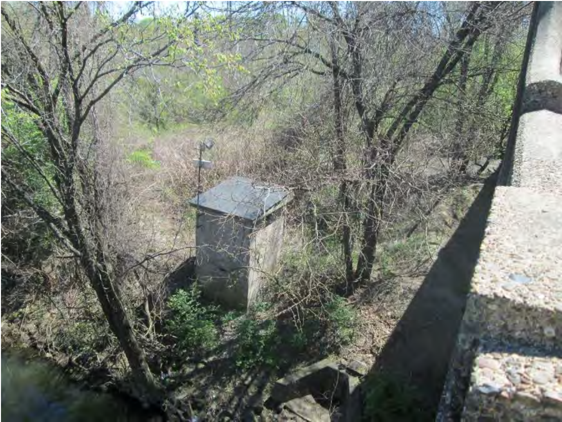
Figure 29 – Assunpink Creek USGS Station and Headwall, looking northeast
