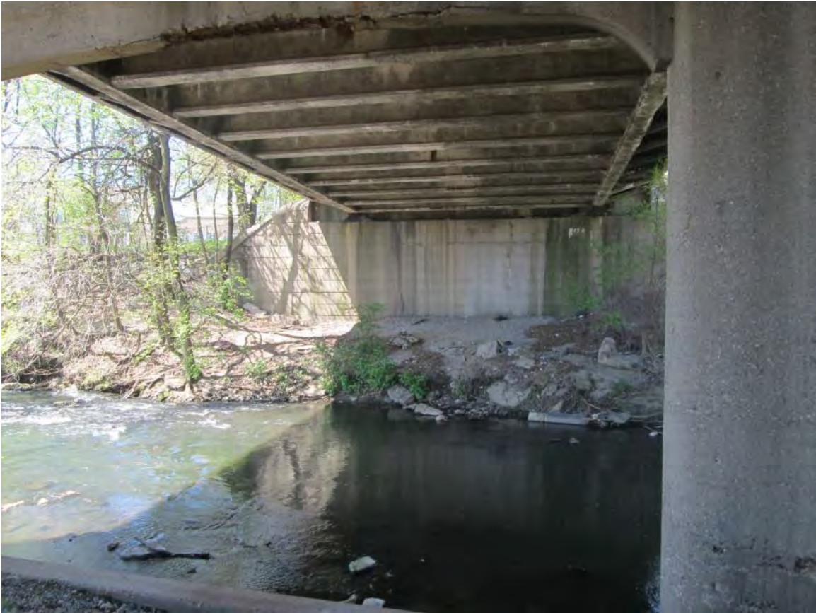
Figure 17 – Pier 7, looking west at Western Abutment
