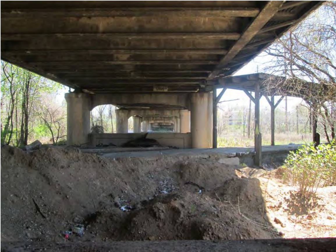
Figure 13 – Piers 1-5 and Inactive NJ Transit Station Platform, looking east
