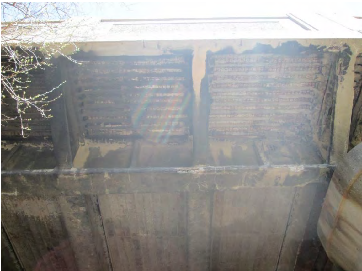
Figure 10 – Underside of sidewalk, showing 10 existing conduits
