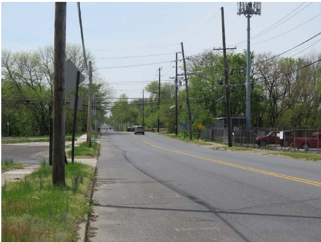
Plate 6: Western approach of the Kaighns Avenue Bridge.
