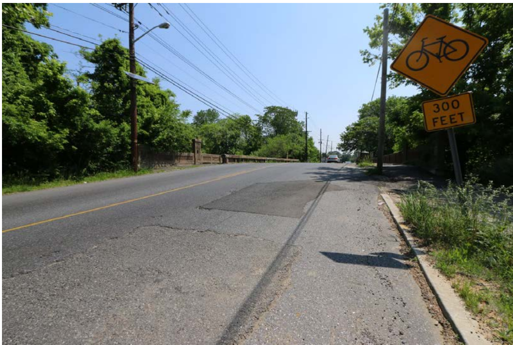
Plate 4: Eastern approach of the Kaighns Avenue Bridge.
