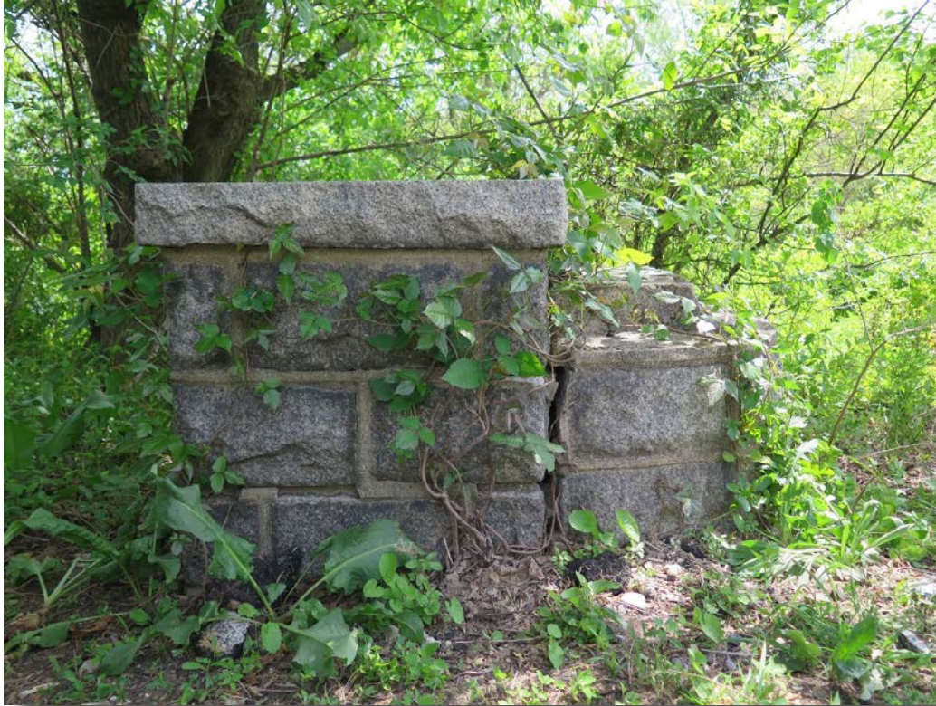
Plate 15: Remnants of a stone staircase adjacent to the Kaighns Avenue Bridge.
