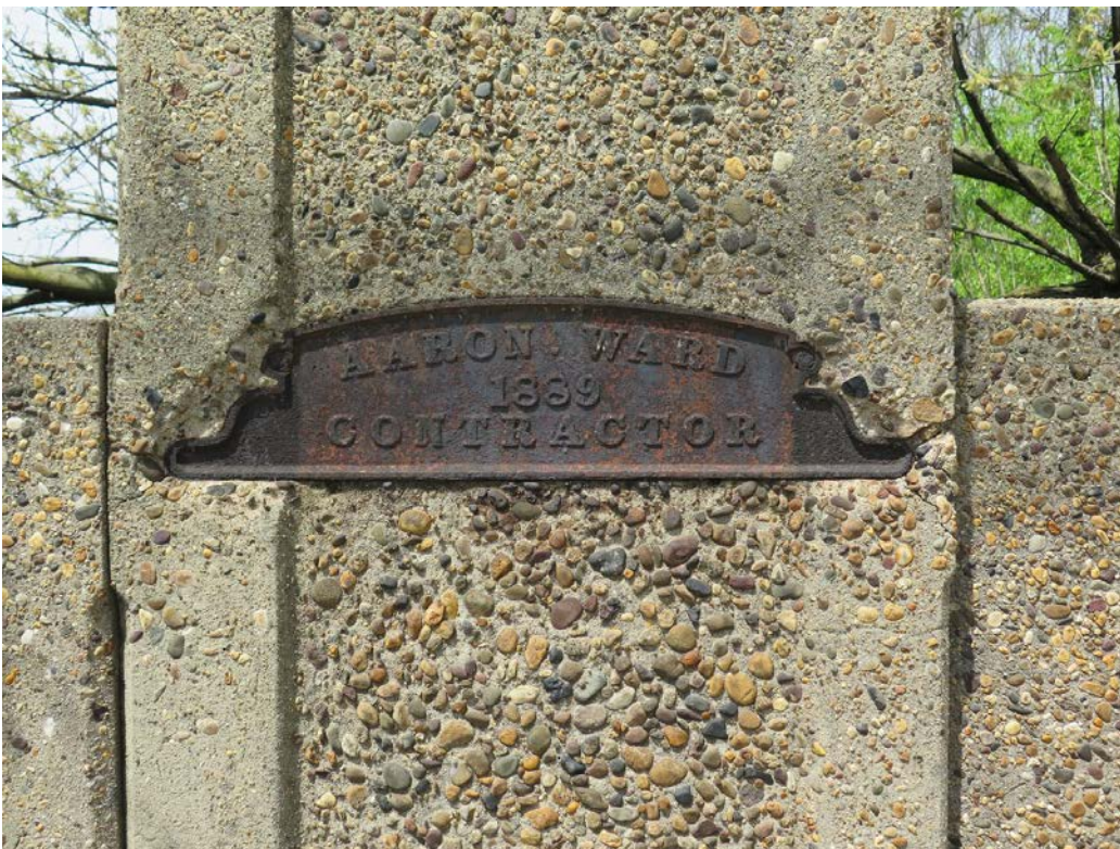
Plate 14: A circa 1889 Aaron Ward contractor plate that predates the bridge.
