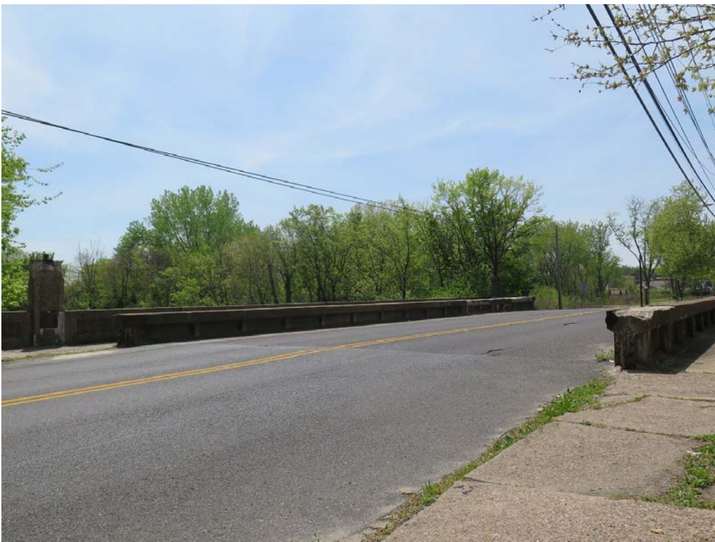
Plate 2: View of the Kaighns Avenue Bridge.
