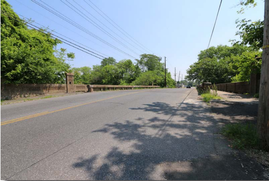
Plate 1: Eastern approach of the Kaighns Avenue Bridge.
