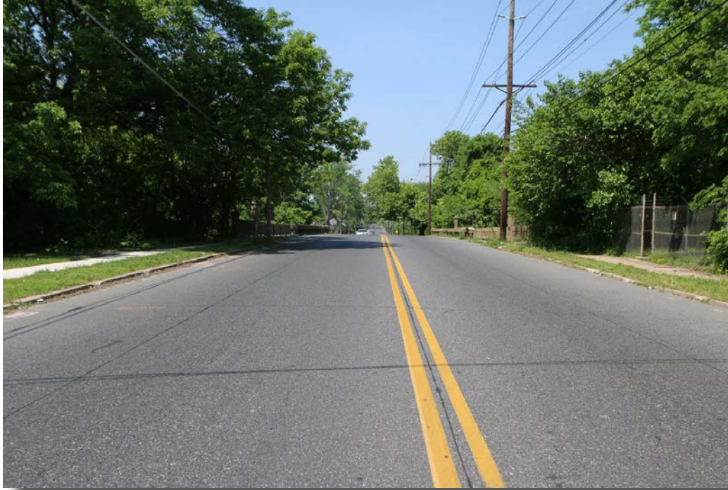
Plate 7: Western approach of the Kaighns Avenue Bridge.
