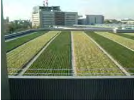
Rooftops can provide ideal locations for sustainable agriculture in urban locations and also help to reduce stormwater runoff.
