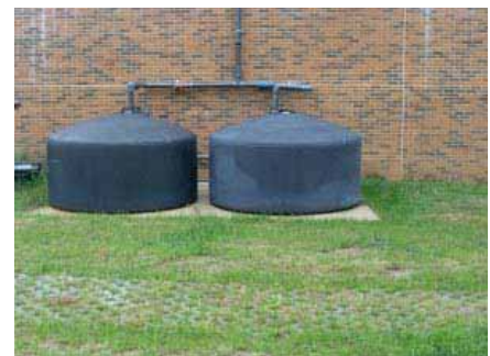
Walnut Hill Community Farm captures water from Septa's 46th St. station roof. With the help of SEPTA's union, they refitted pipes that now run into an 1100 gallon cistern on the site of The Walnut Hill Community Farm. The cistern is then connected to a pipe system that Philly Rooted designed. The pipes run into a mechanical water pump that is hooked up to a car battery, via a power inverter, which is powered by a 15 volt solar panel.
