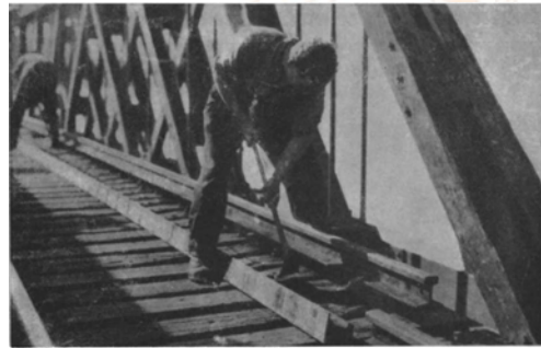
A bridge repair job in progress. (Rtg. Publicity photo.)
