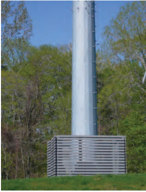
Bergey WindPower 10kW XLS monopole turbine with fence in Erie, PA
