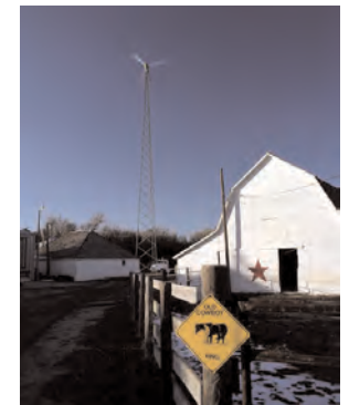
Bergey WindPower 10kW XLS turbine
