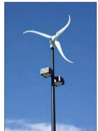
Skystream 1.8kW turbine dual-use on lamppost
