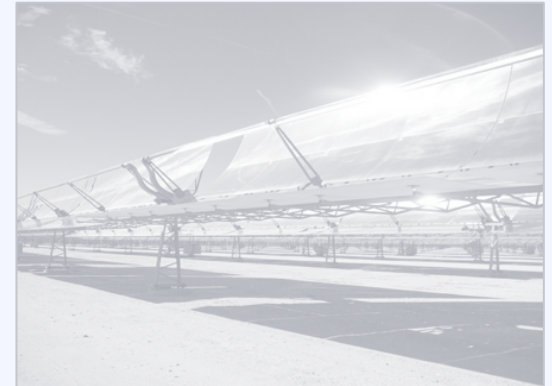
Concentrated Solar Power
