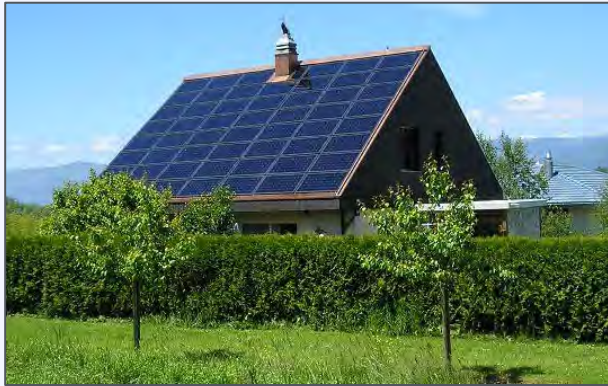
Solar Photovoltaic (PV)
