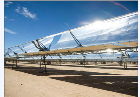
Concentrated Solar Power
