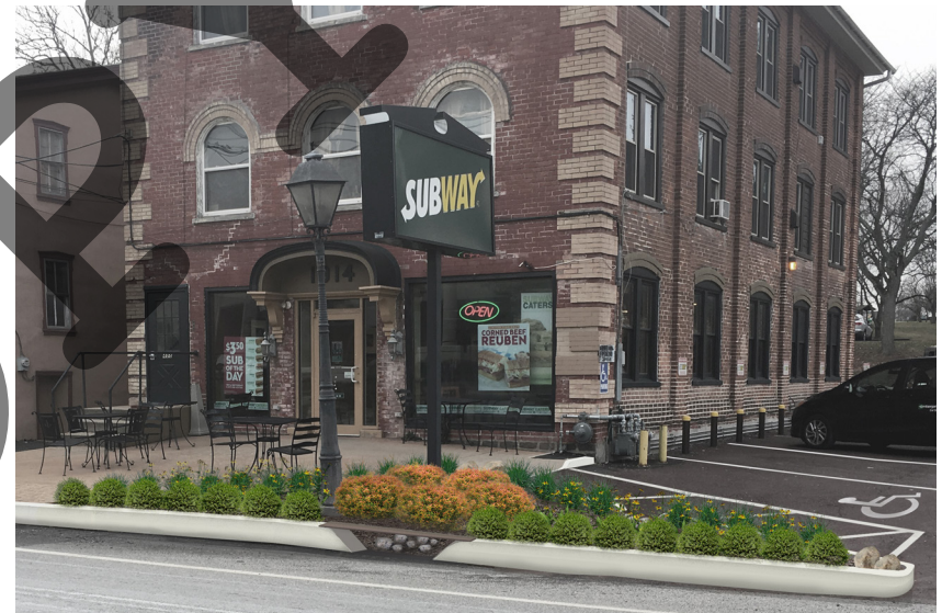
Green Stormwater Infrastructure: AFTER
