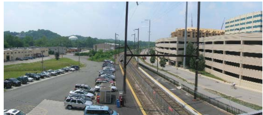
The Conshohocken Station as seen from Fayette St. At its best, a train station is a welcoming experience, a representation of how a town views itself.
