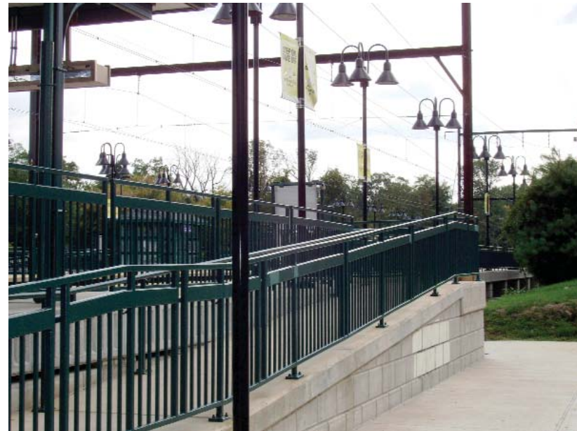
ADA ramp from parking lot to platform at Melrose Park.
