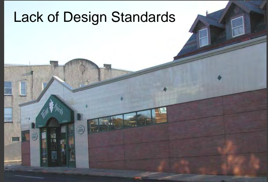
Lack of Design Standards
