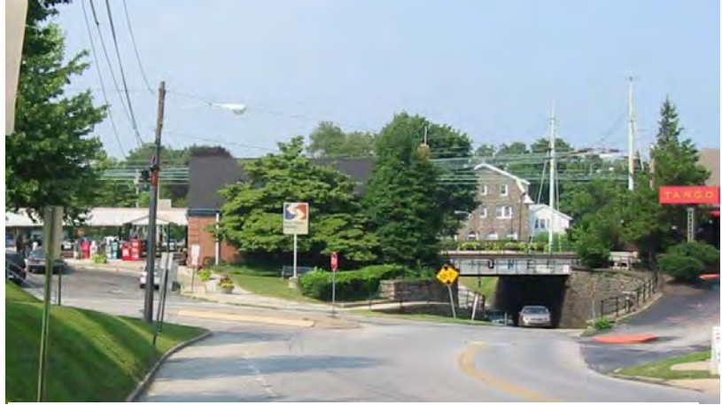
Figure 3: Railroad Corridor Crossing
