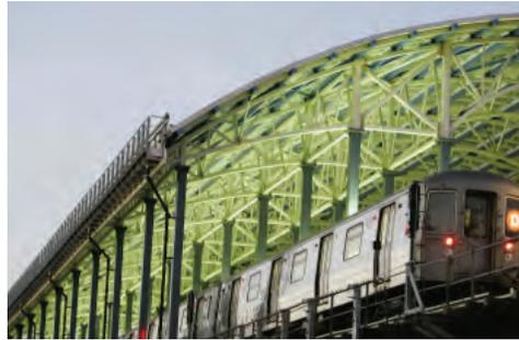
Stillwell Avenue/Coney Island Terminal rebuilt with a roof made up of photovoltaic solar cells
