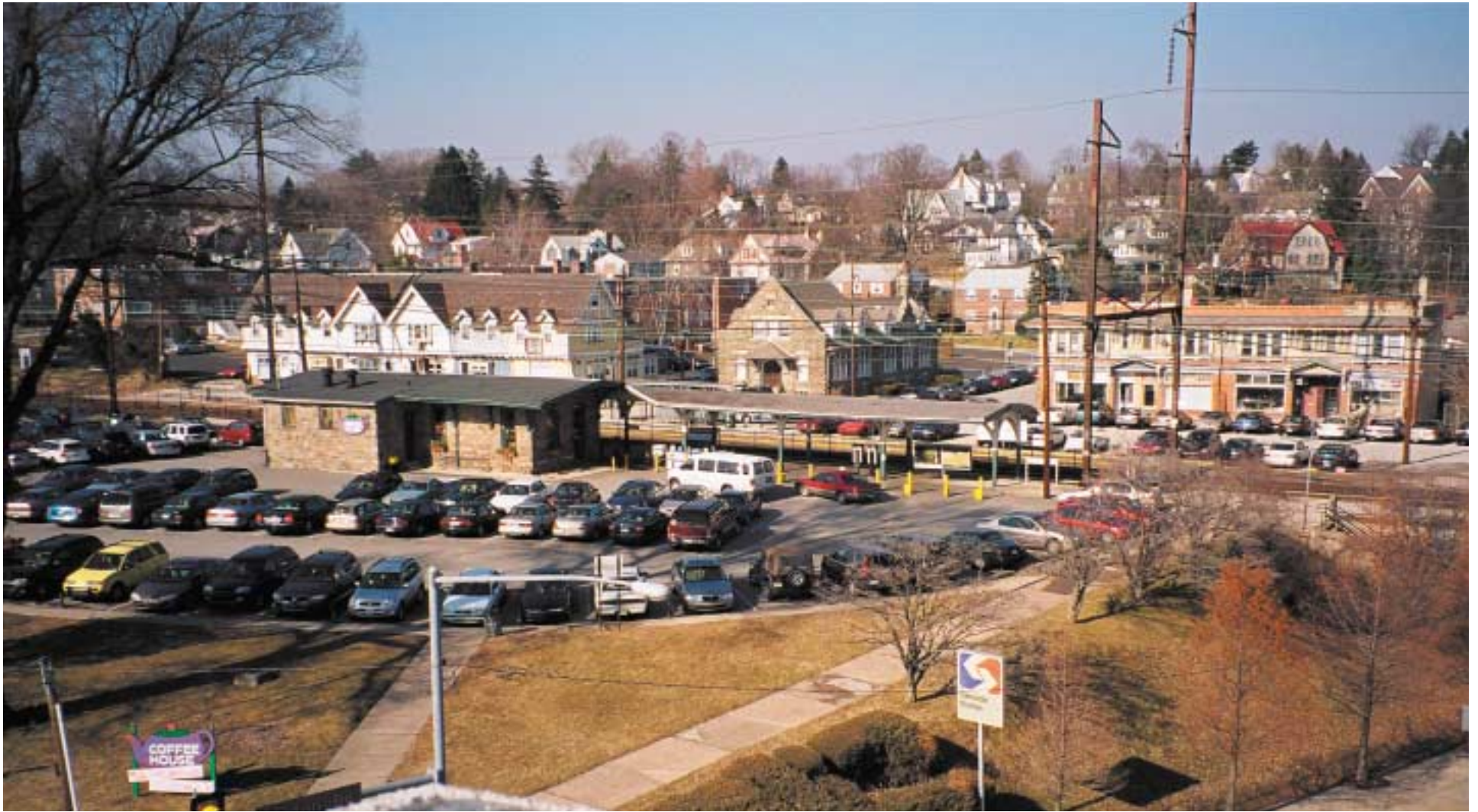
figure 2.1.0 Aerial View of Glenside Station and Roberts Block
