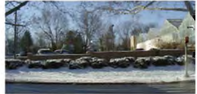
Knee Wall at Parking Lot
