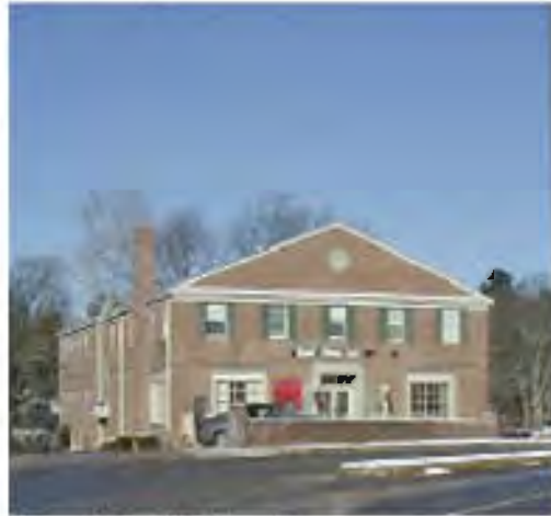
Knee Wall at Parking Lot
