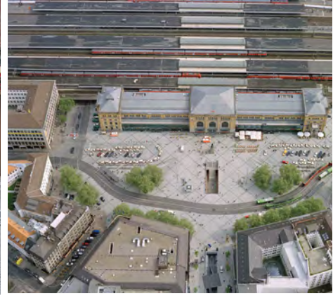
Figure 41 Active Station Plaza, Hanover, Germany
