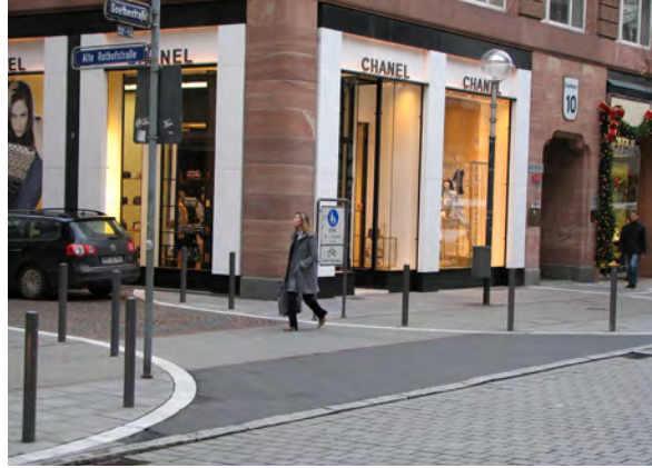
Figure 40 Road Surface Raised to Pedestrian Level
