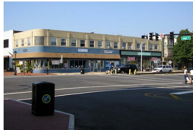
Photo 9. Bump-outs at High and Broad Street Crosswalk.
