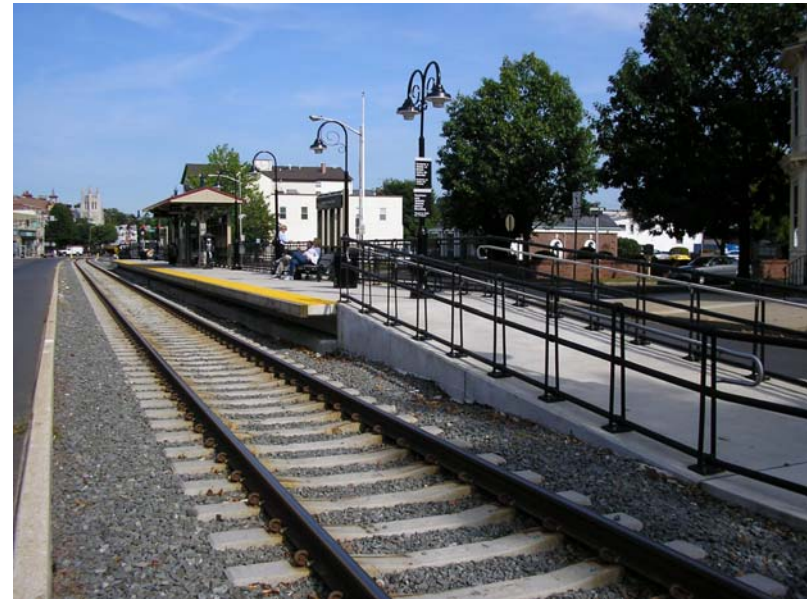
Photo 8. Light Rail Station on Broad Street
