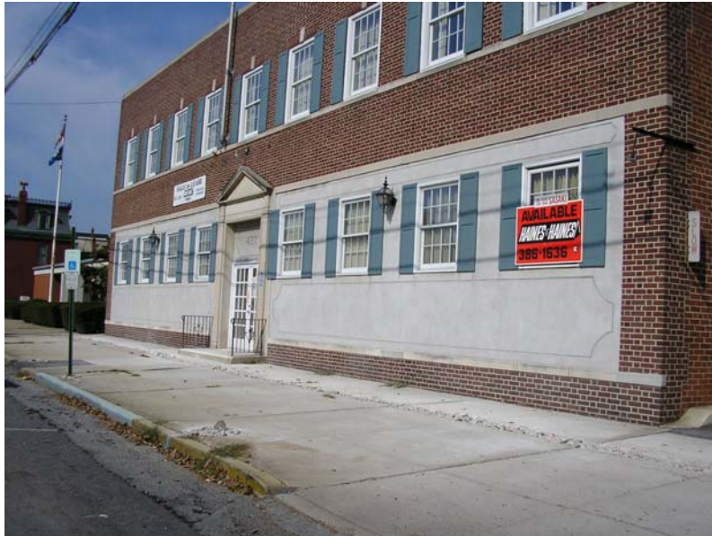
Photo 3. Vacant former City Hall offices at 437 High Street in C-1 Zone
