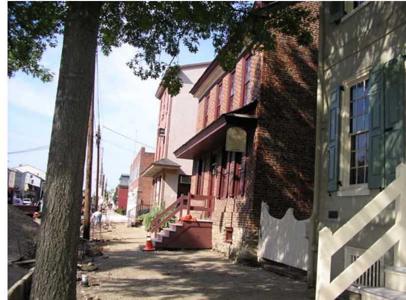
Photo 10. 400 Block High Street under Construction
