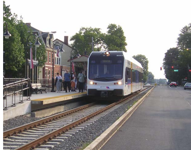
Photo 1. Burlington Towne Center Light Rail Station
