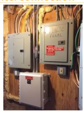
At the location of the ground-fault protection, normally at the inverter, warning of a shock hazard (*NEC* 690.5[C]).
