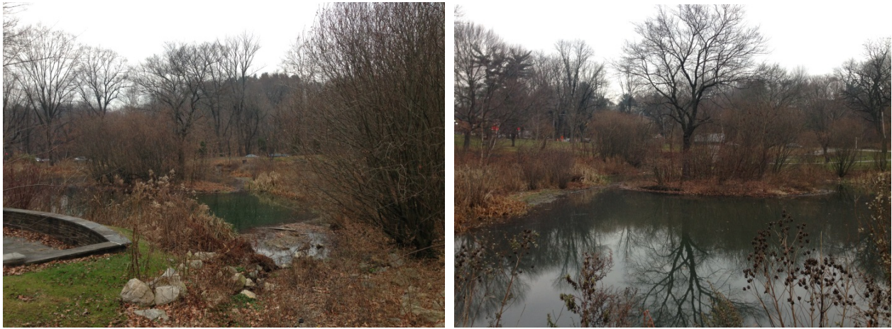
Figure 5. Saylor's Grove stormwater treatment wetland, Philadelphia, PA.
