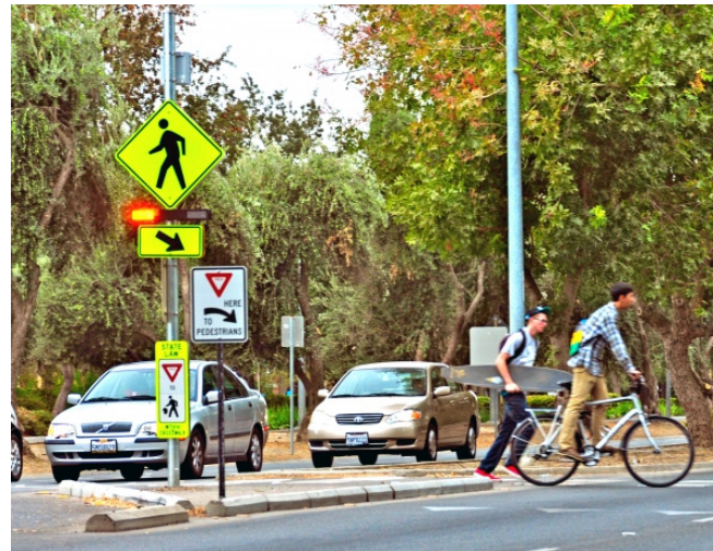
Rectangular Rapid Flashing Beacon (RRFB) in Davis, CA Source: www.pedbikeimages.org / Lara Justine
