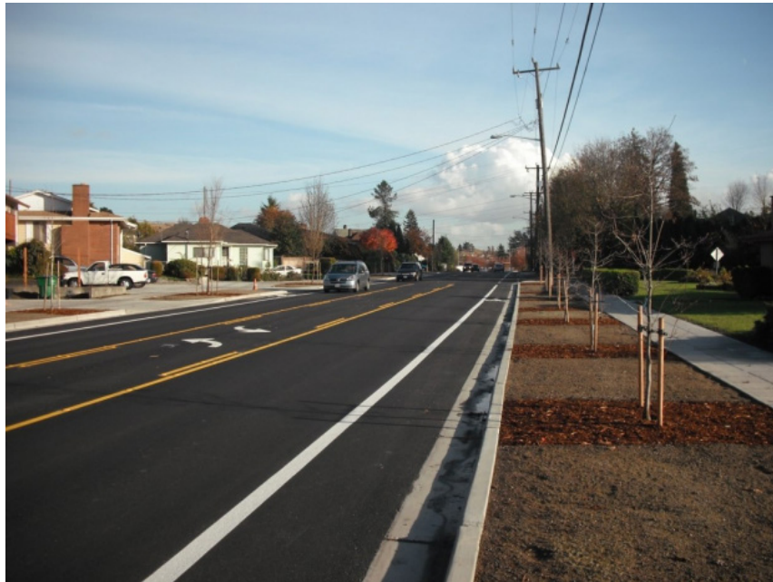
Road Diet in Santa Barbara, CA Source: www.pedbikeimages.org
