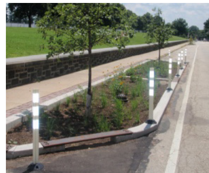
Stormwater Bumpout, Philadelphia
