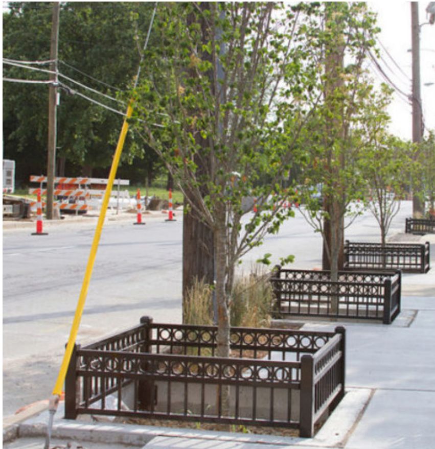
Stormwater Tree Pits in Louisville, KY Source: NACTO
