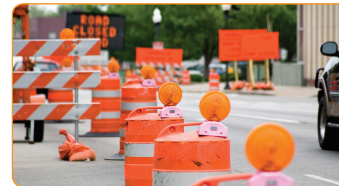
A typical work zone set-up in southeastern Pennsylvania
