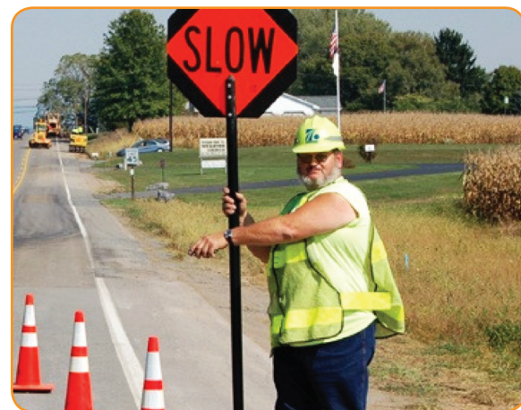
Example of proper flagging technique (Courtesy of PennDOT LTAP)
