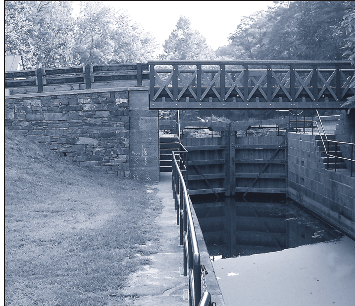
The Schuylkill Navigation Lock in Upper Providence Township, Montgomery County, is a Transportation Enhancement project which was recently completed. Restoration of the 1846 canal included removing fill at one end, replacing it with a historically accurate truss bridge, installing mitre gates at both ends, and reproducing the original toll house. The Locktender's House will also be restored as a community and visitor's center.
