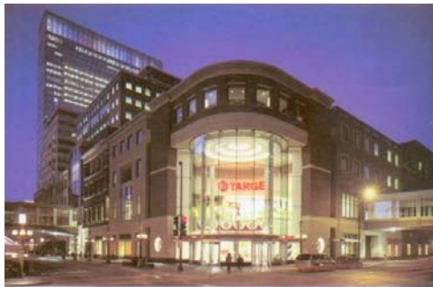
This four-story Target in downtown Minneapolis, MN is pedestrian-friendly and designed to match its urban context. Source: APA / Target Corporation
