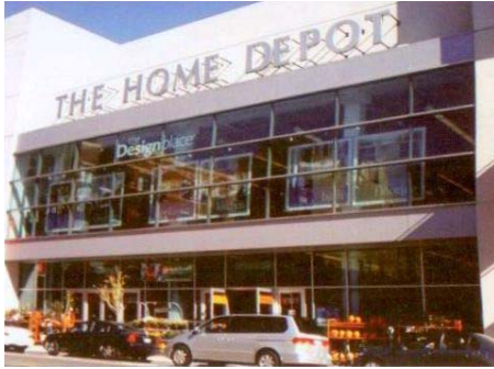
This Home Depot in Lincoln Park, Chicago fits well with its urban setting. Source: APA / Jonathan Mendel
