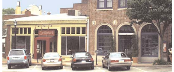
In Radnor Township, Pennsylvania, portions of the Wayne commercial area comprise a registered historic district.
