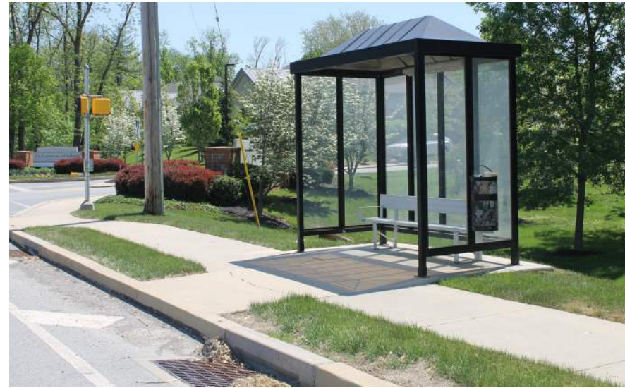
Figure 19: Waiting Area with Standard Shelter
