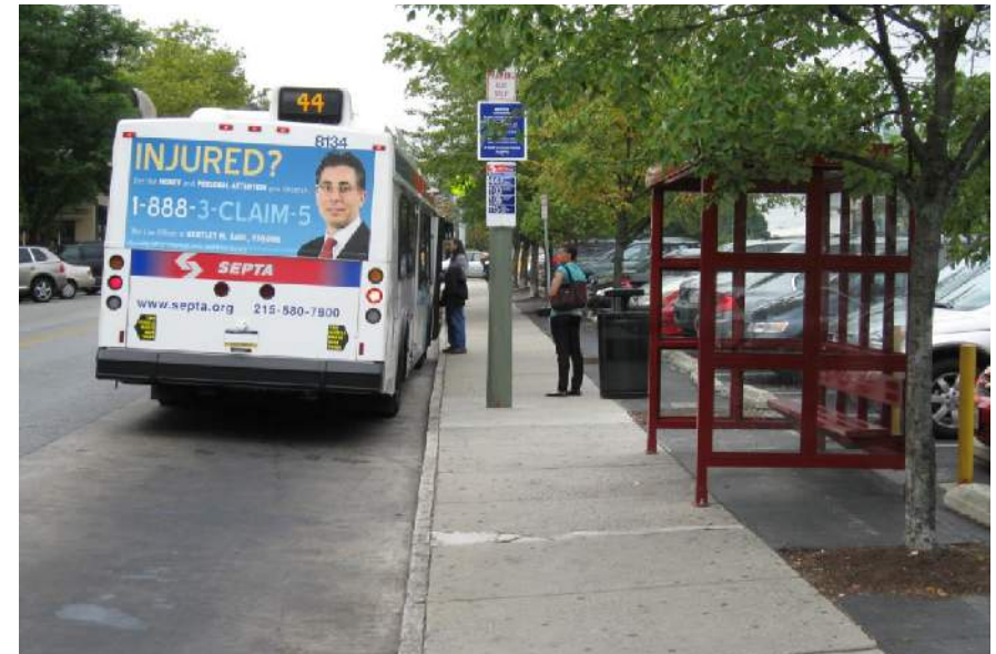
Figure 13: Concrete Pad in Street at Bus Stop Area, Ardmore, PA
