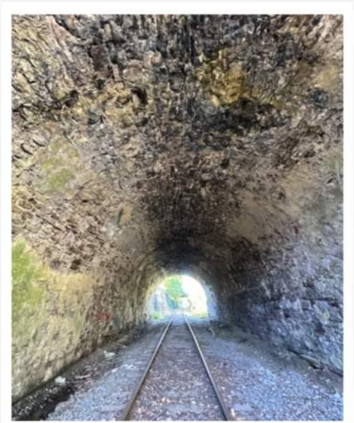
Bordentown Stone Arch Bridge (11/2022)
