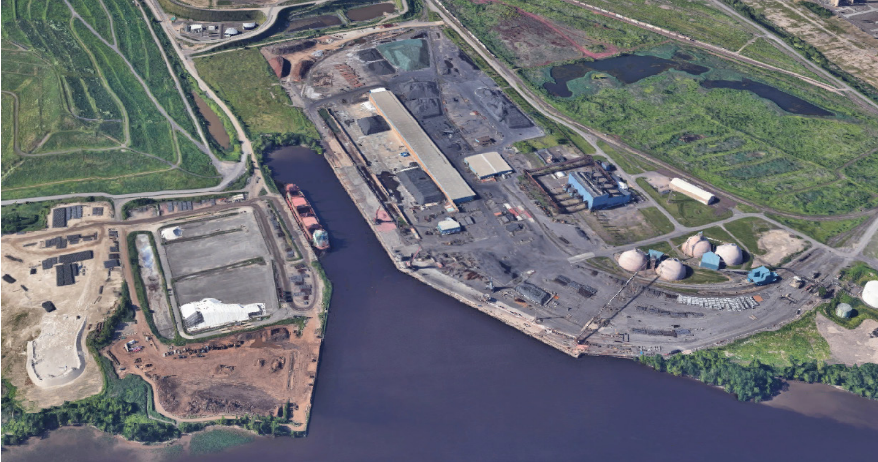
Aerial Image of the Fairless Hills Marine Terminal (Left) and the Port of Bucks (Right). Source: Google (2023)
