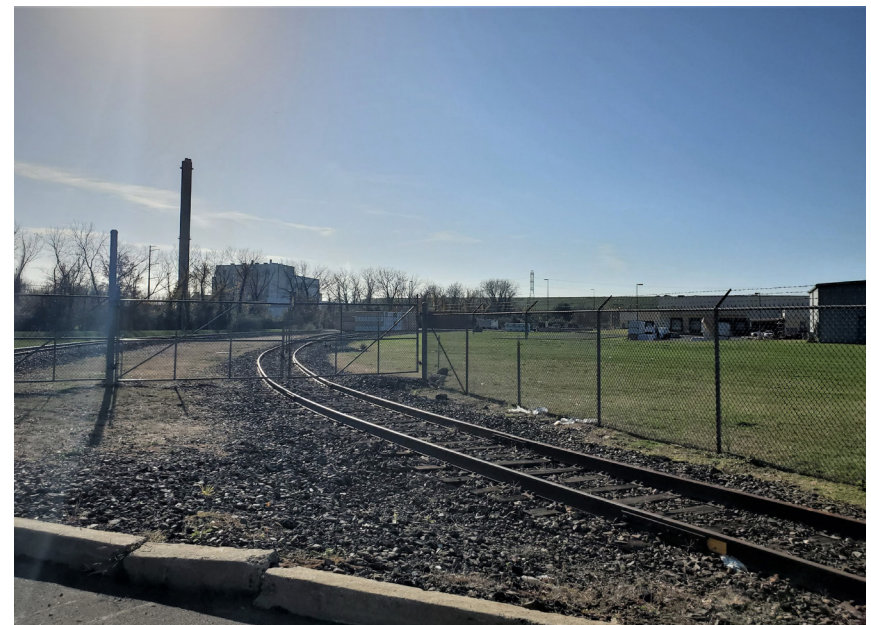
Rail Access to an Existing Facility in the KTC.
