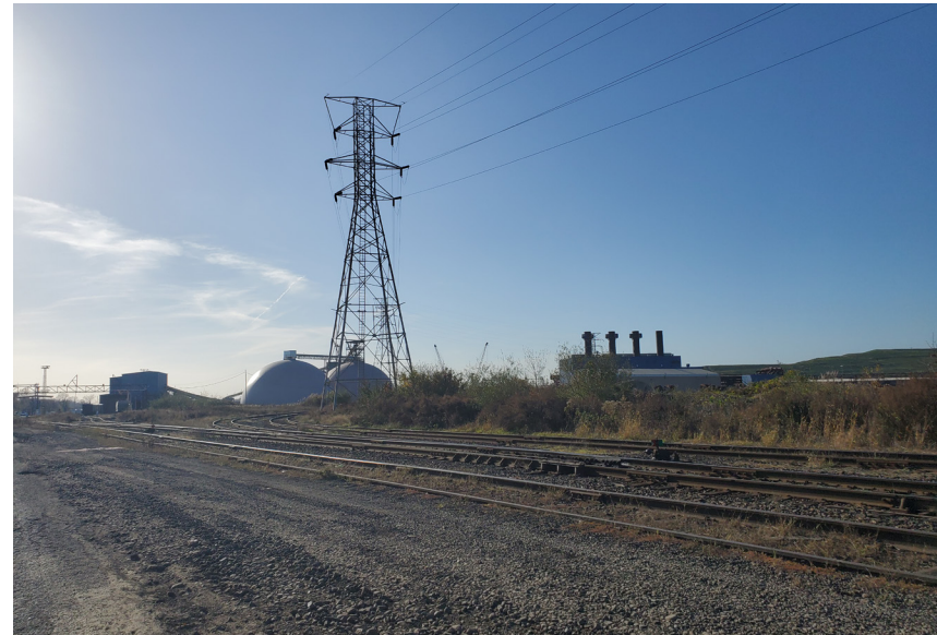
Existing High Voltage Transmission Lines Within the KTC.
