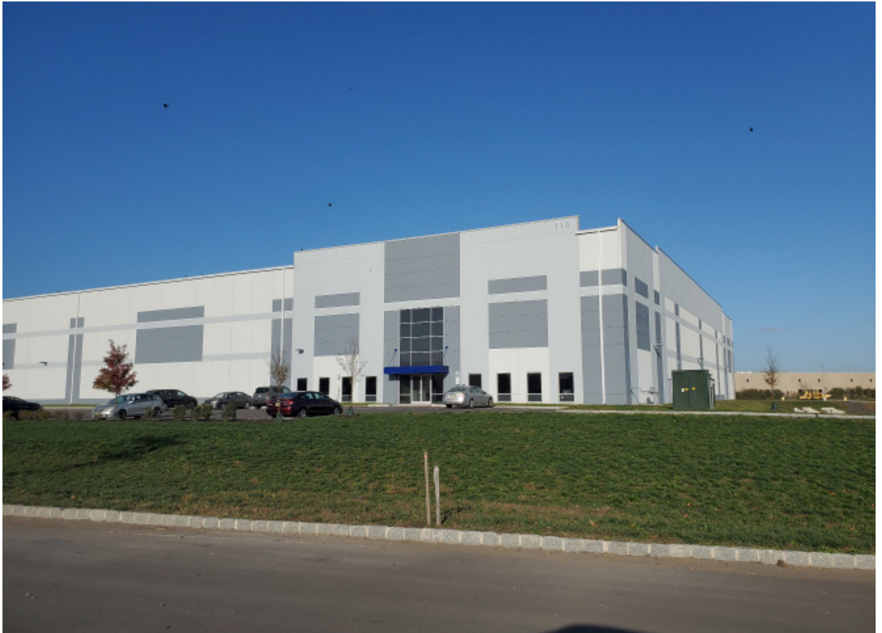
Recently Completed Phase 1 Distribution and Logistics Space in the KTC. Source: DVRPC
