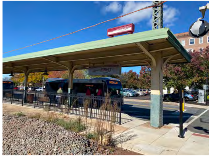
Charles W. Dickinson Transportation Center Source: DVRPC (2021)
