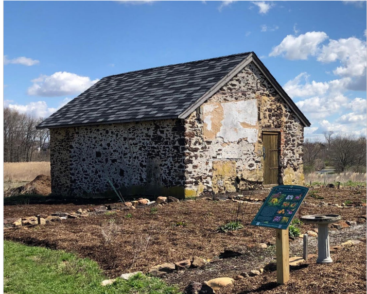
Barn at Swede Run Fields
